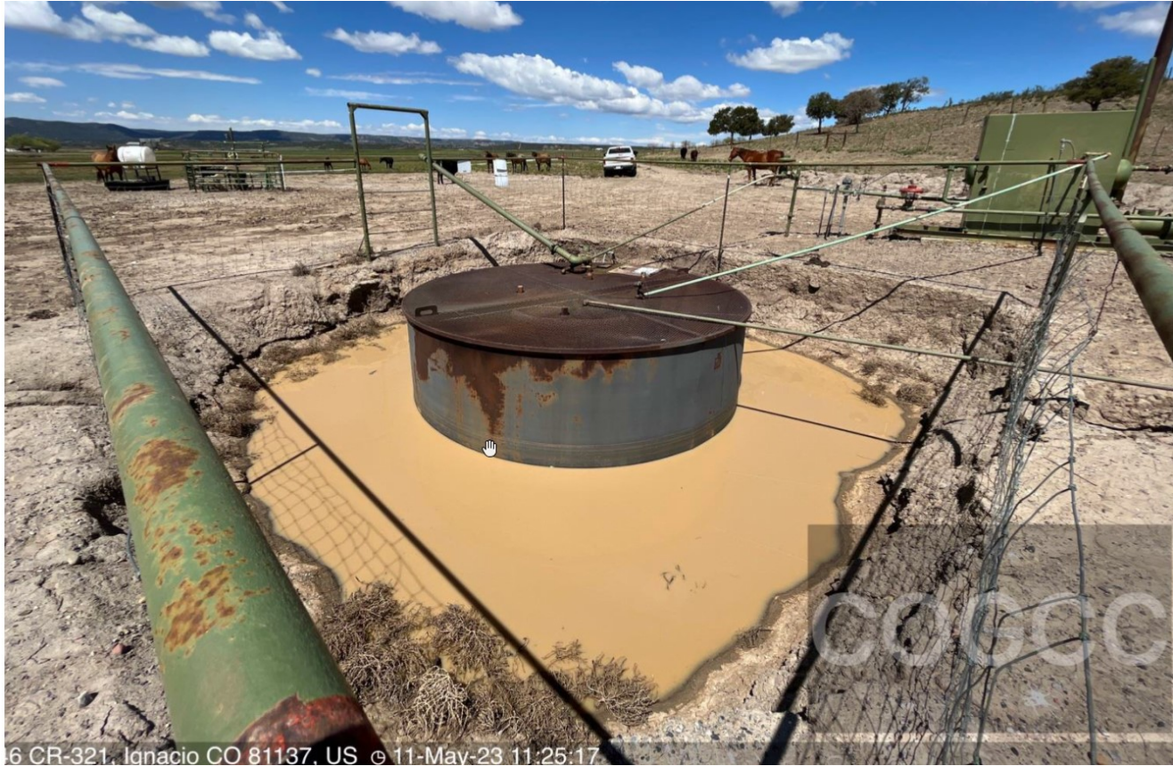
Picture from INC showing the containment around the pit with water in it.
