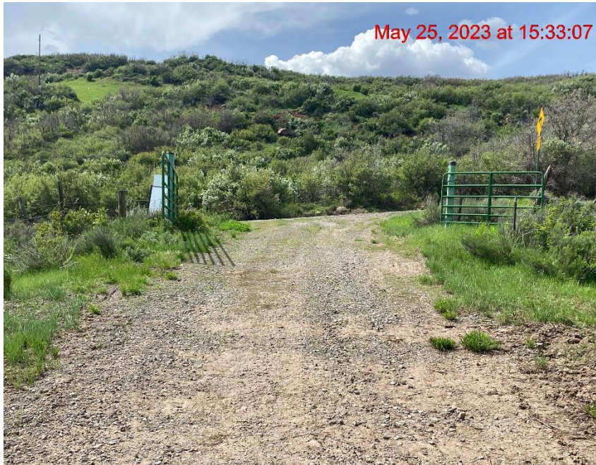
Insufficient Vehicle Tracking BMPs at Location Entrance/Exit – Photo #03913
