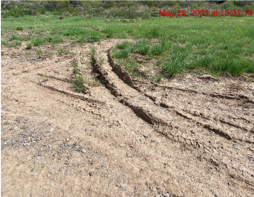
Location Lacks Stabilization – Photo #03909
