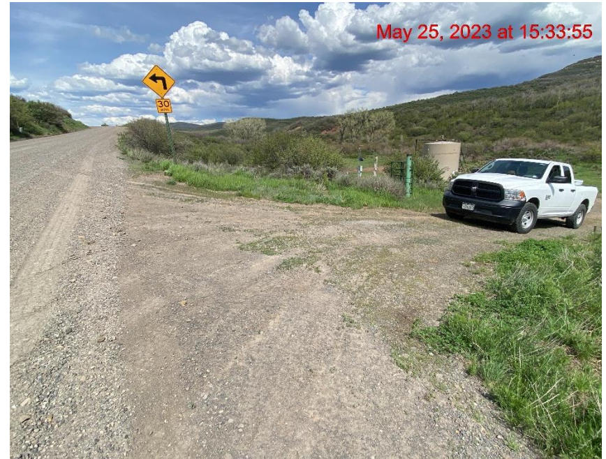
Insufficient Vehicle Tracking BMPs at Location Entrance/Exit – Photo #03914
