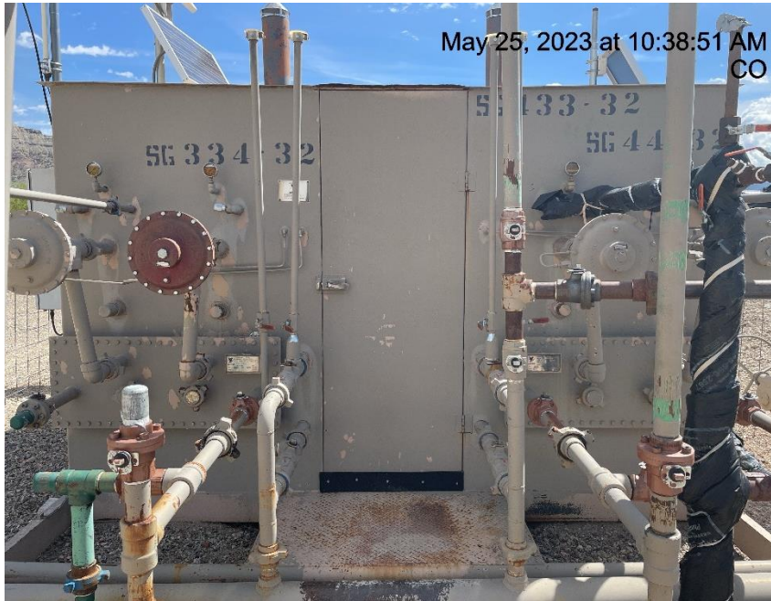
Photo # 8784 Meter calibration info not conspicuously posted
