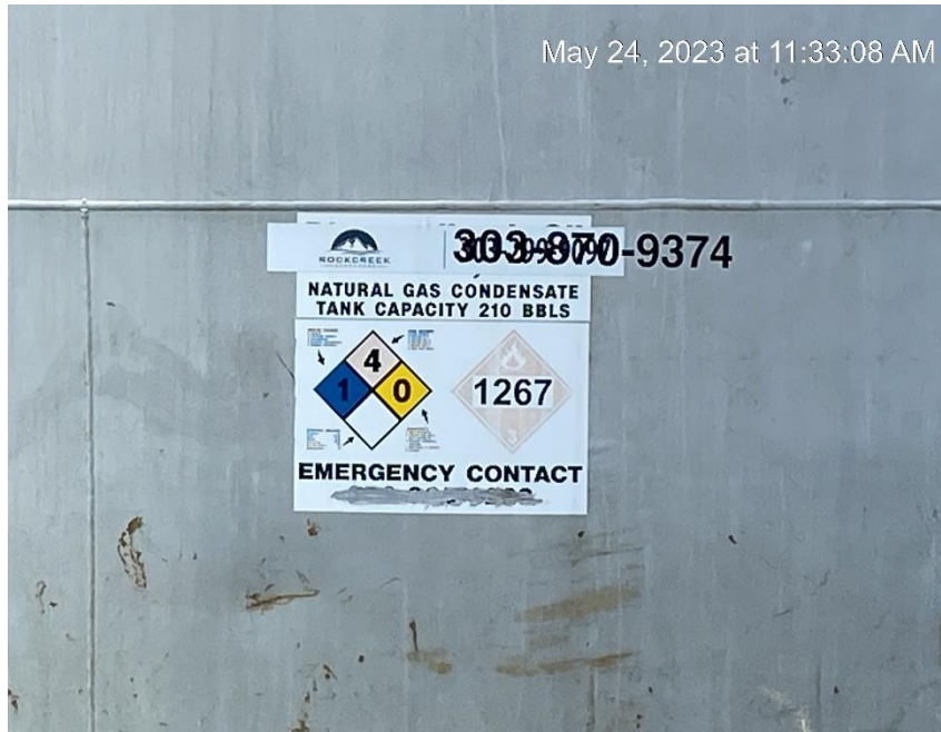
Tank lacking required information
