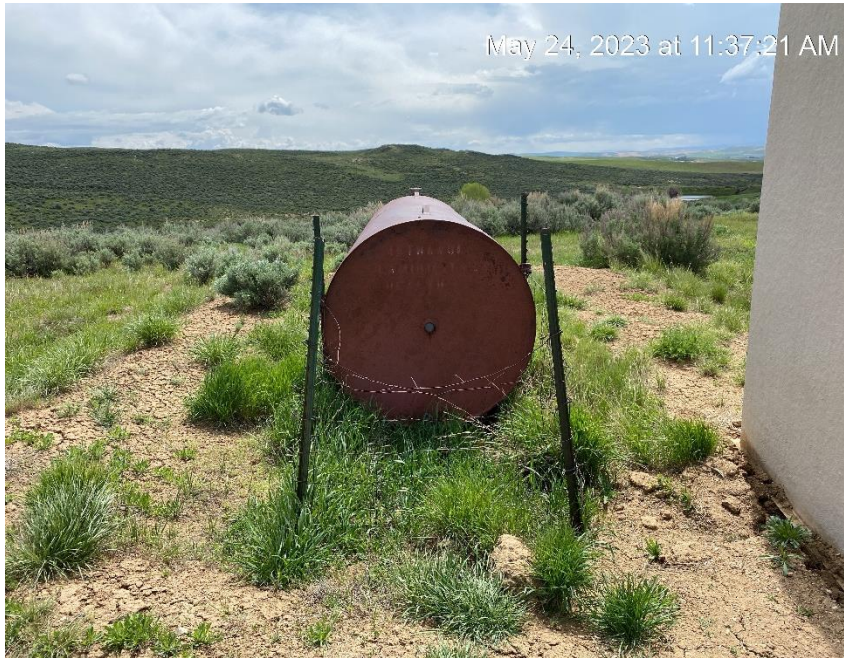
Tank not labeled. Not in proper containment
