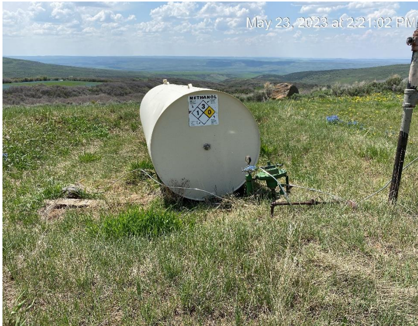
Methanol tank not in sufficient containment
