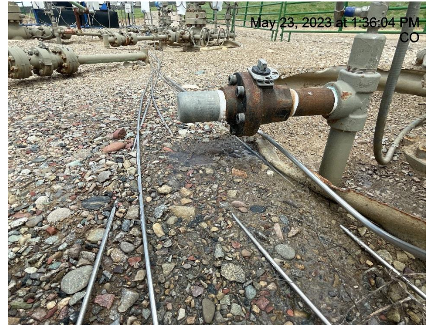
Photo # 8436 Valve on bradenhead leaking fluid onto ground
