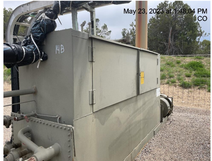
Photo # 8474 Meter calibration info not conspicuously posted
