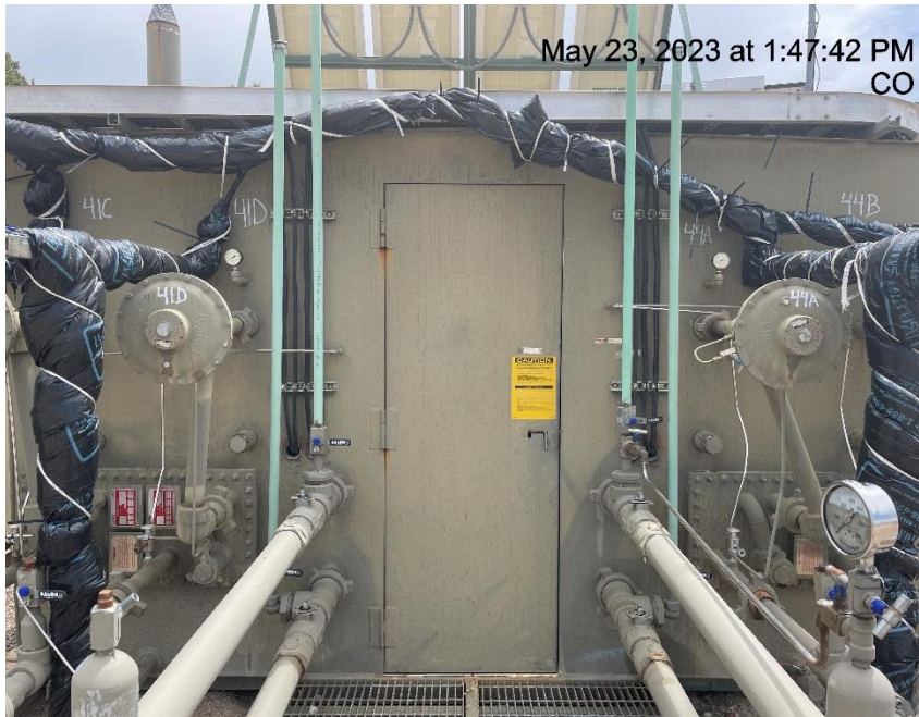
Photo # 8471 Meter calibration info not conspicuously posted
