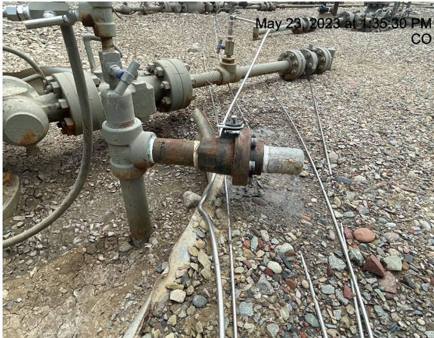
Photo # 8433 Valve on bradenhead leaking fluid onto ground
