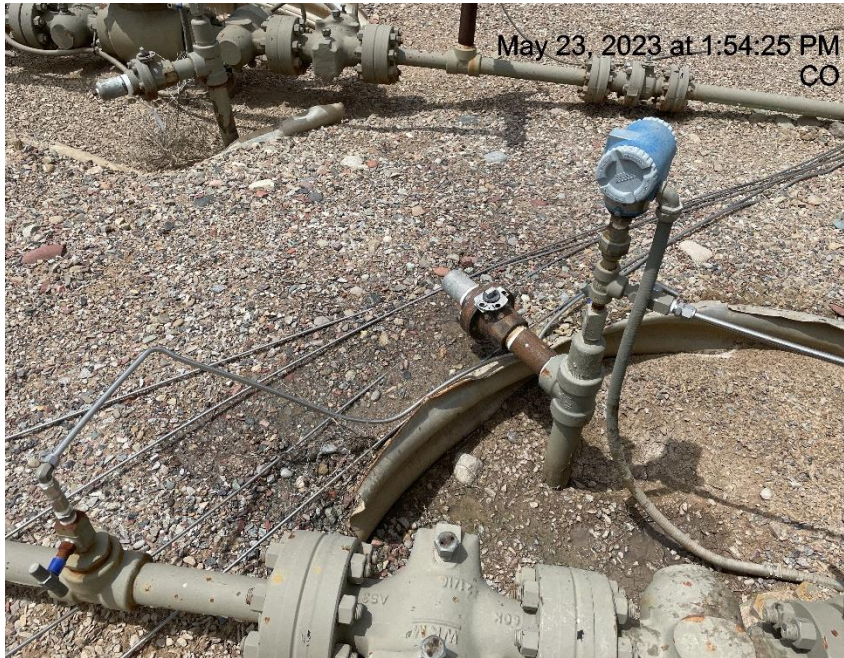
Photo # 8481 Valve on bradenhead leaking fluid onto ground
