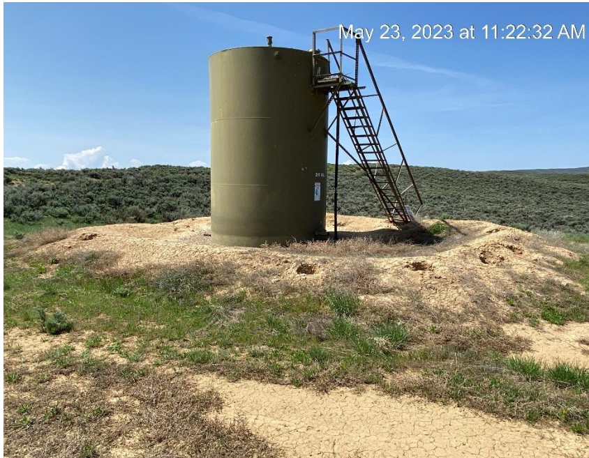
24' x 25' berm inadequate
