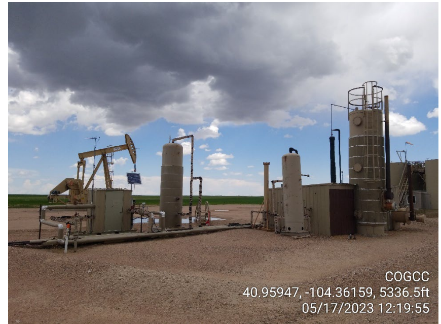
Photo 8 – Gas Meter and Heater Treater
