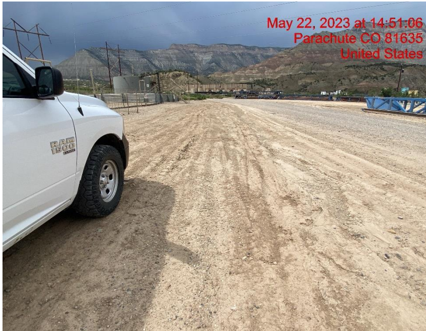
Insufficient Vehicle Tracking BMPs at Location Entrance/Exit – Photo #03669
