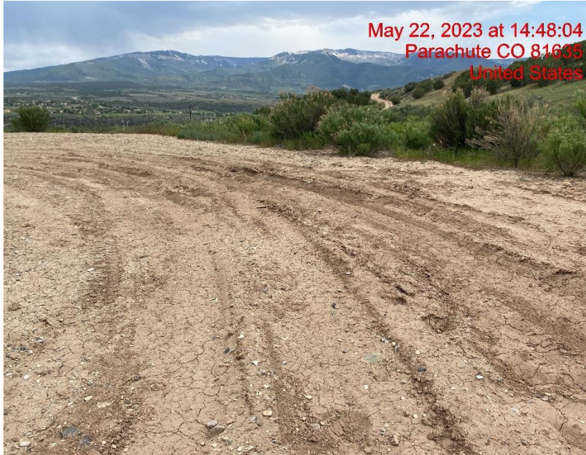
Location Lacks Stabilization – Photo #03661
