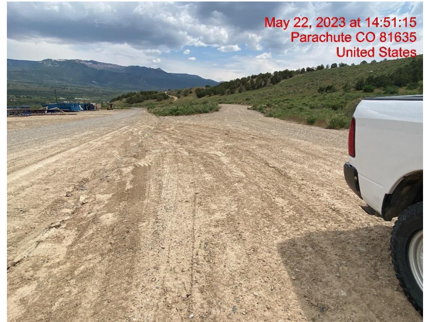
Insufficient Vehicle Tracking BMPs at Location Entrance/Exit – Photo #03670
