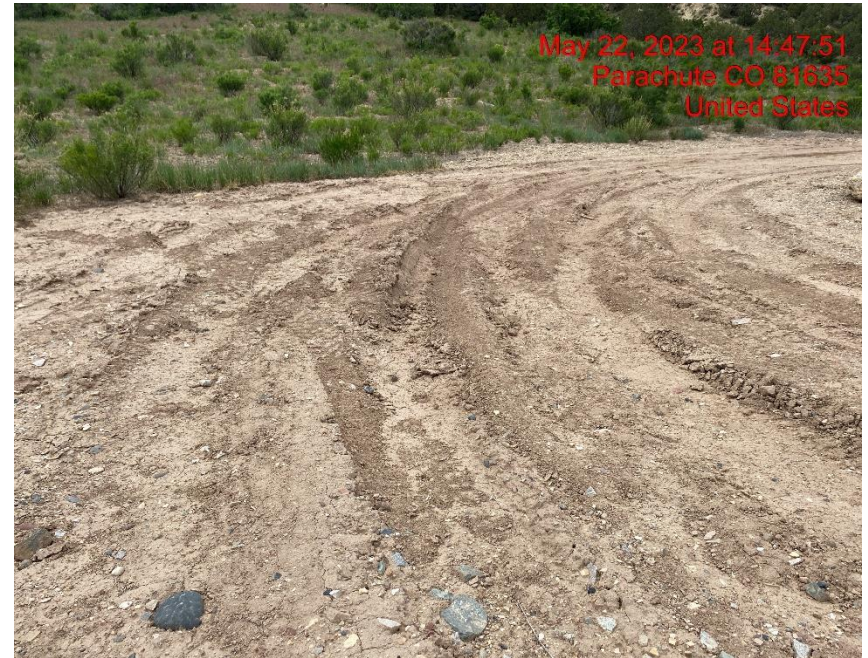
Location Lacks Stabilization – Photo #03660
