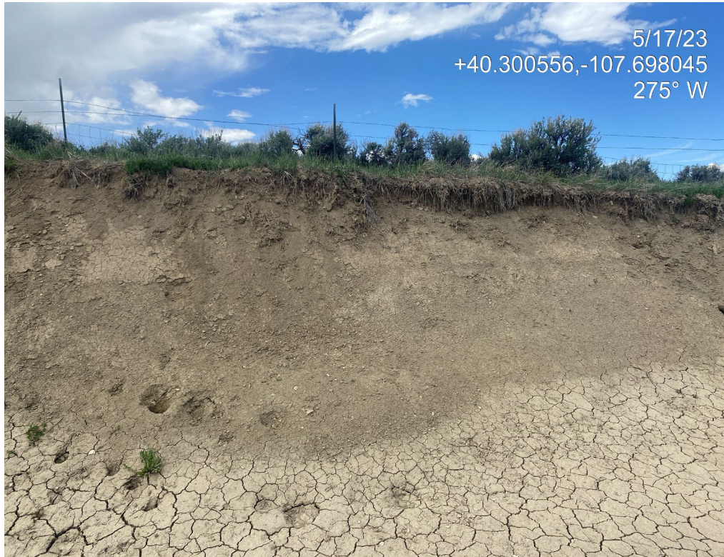
Photo 8. Photos show the cut slope is unstable. Vegetation is pedestaled with exposed roots. Erosion appears to be migrating upslope/backwards, undercutting into undisturbed reference areas. Rill erosion is occurring.
