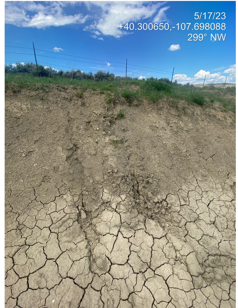
Photo 8. Photos show the cut slope is unstable. Vegetation is pedestaled with exposed roots. Erosion appears to be migrating upslope/backwards, undercutting into undisturbed reference areas. Rill erosion is occurring.
