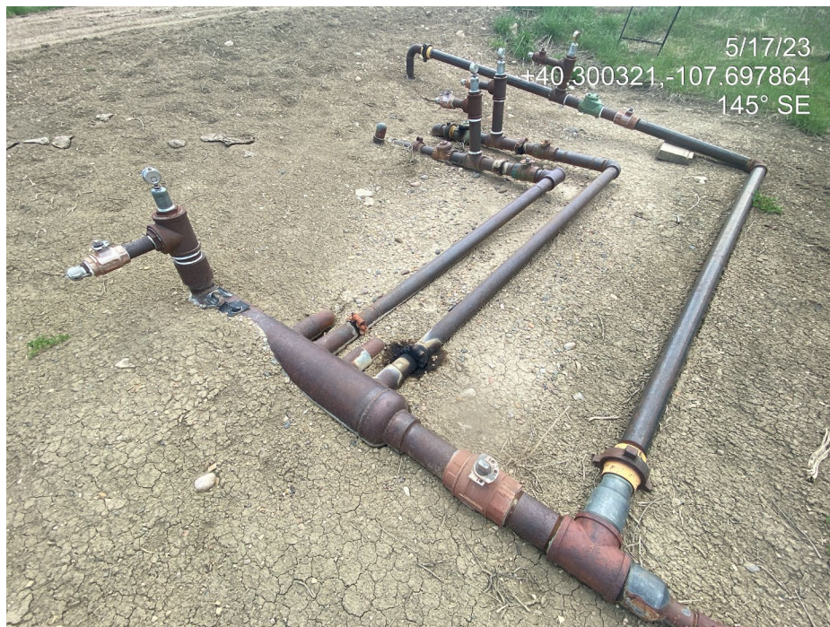
Photo 4. Photos show staining at the cathodic protection unit.
