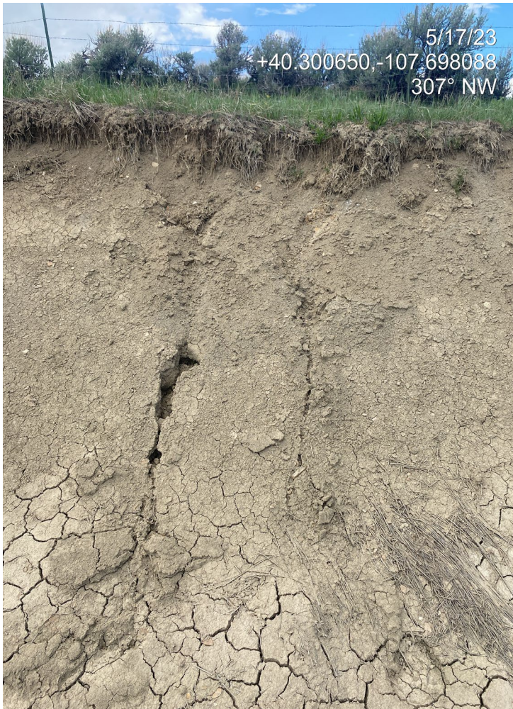
Photo 7. Photos show the cut slope is unstable. Vegetation is pedestaled with exposed roots. Erosion appears to be migrating upslope/backwards, undercutting into undisturbed reference areas. Rill erosion is occurring.
