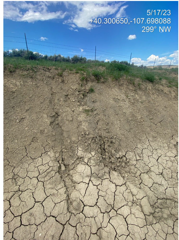
Photo 7. Photos show the cut slope is unstable. Vegetation is pedestaled with exposed roots. Erosion appears to be migrating upslope/backwards, undercutting into undisturbed reference areas. Rill erosion is occurring.
