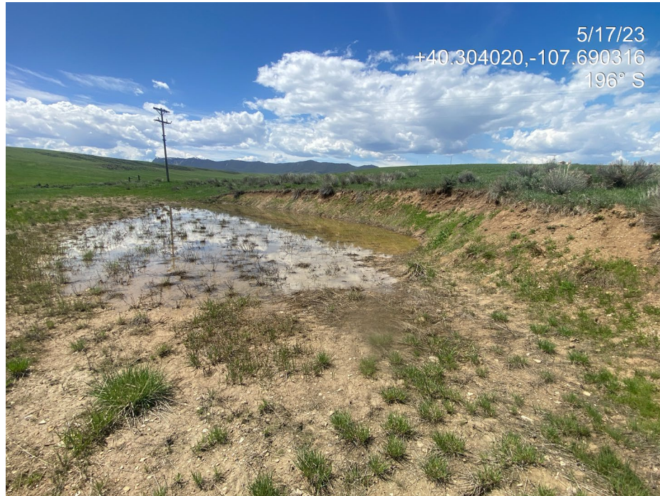
Photo 2. Photos show the location has not been recontoured, an unstabilized cut slope, and lack of vegetation establishment.
