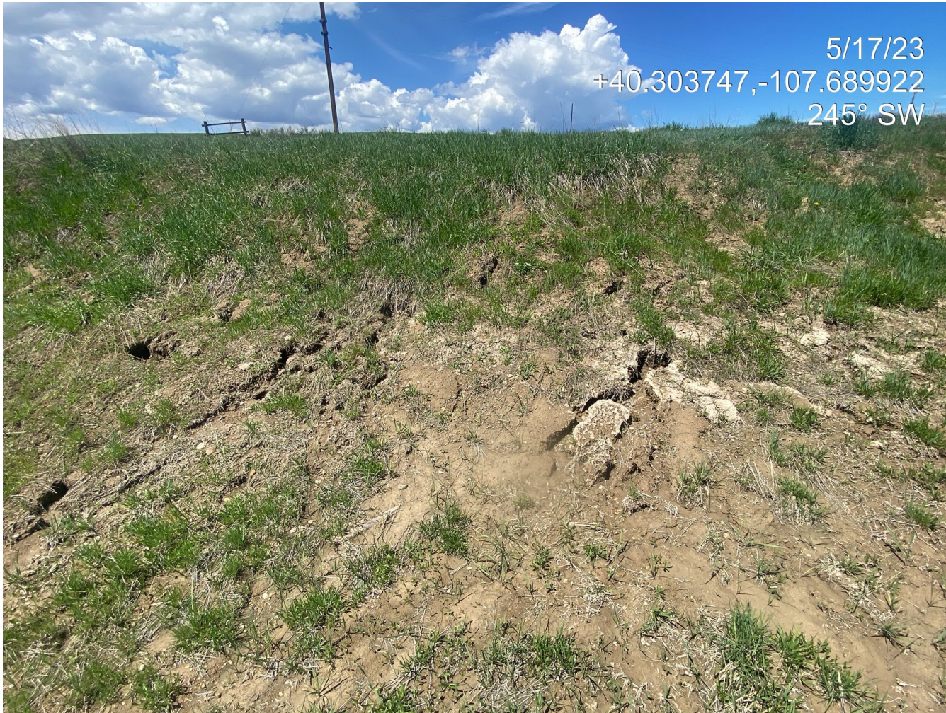
Photo 4. Photo shows erosion in the fill slope.
