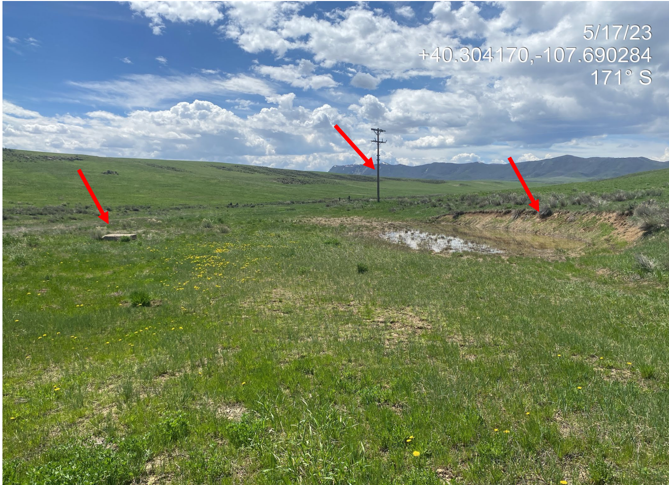
Photo 1. Photo taken from the location entrance to the northwest shows an overview of the location. Note concrete slab, unstabilized cut slope and power line.
