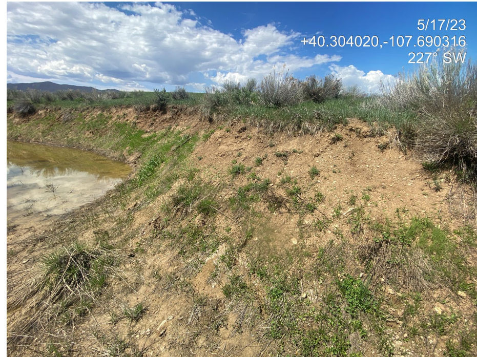
Photo 2. Photos show the location has not been recontoured, an unstabilized cut slope, and lack of vegetation establishment.
