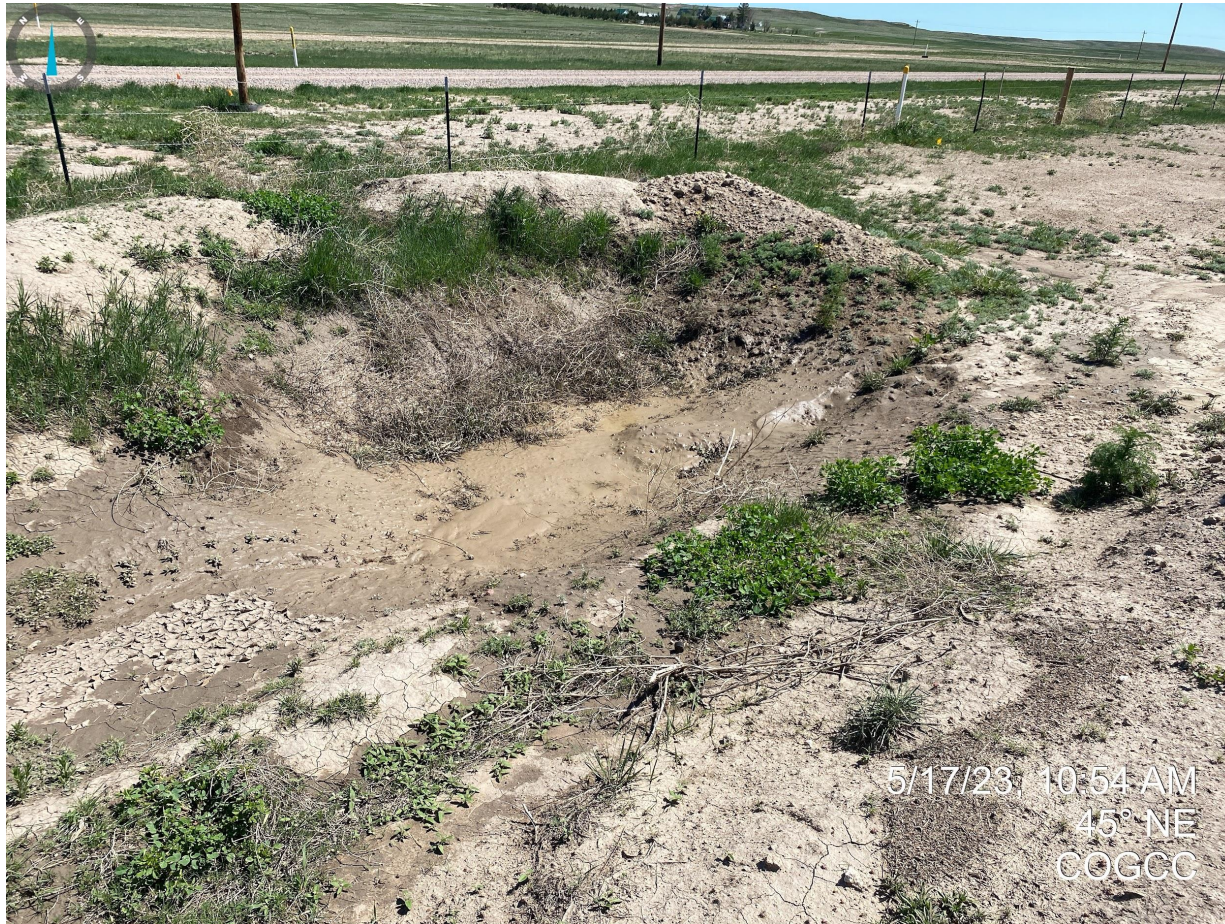
Photo 2. Facing northeast at sediment trap on the northern end of the location. See comments in Photo 1.
