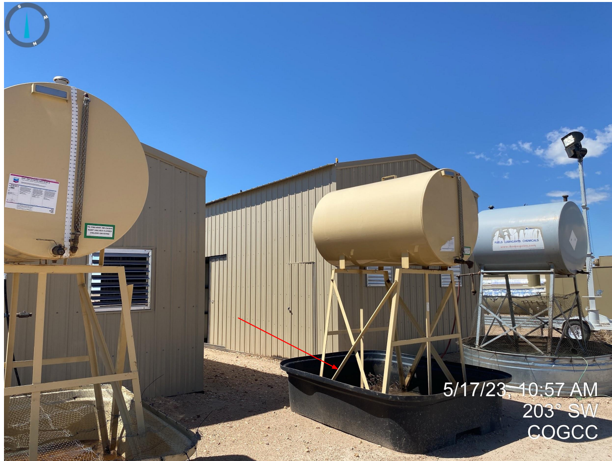
Photo 6. Middle tank did not have any netting installed to prevent wildlife entry.
