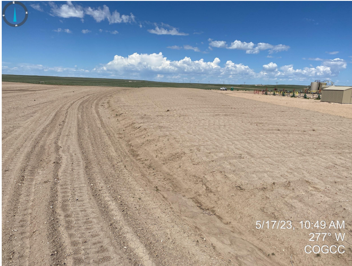
Photo 7. Facing west at the interim reclamation area and topsoil stockpile. Stockpile had evidence of equipment tracking for short term stabilization. The Operator shall continue to comply with interim reclamation timing requirements.
