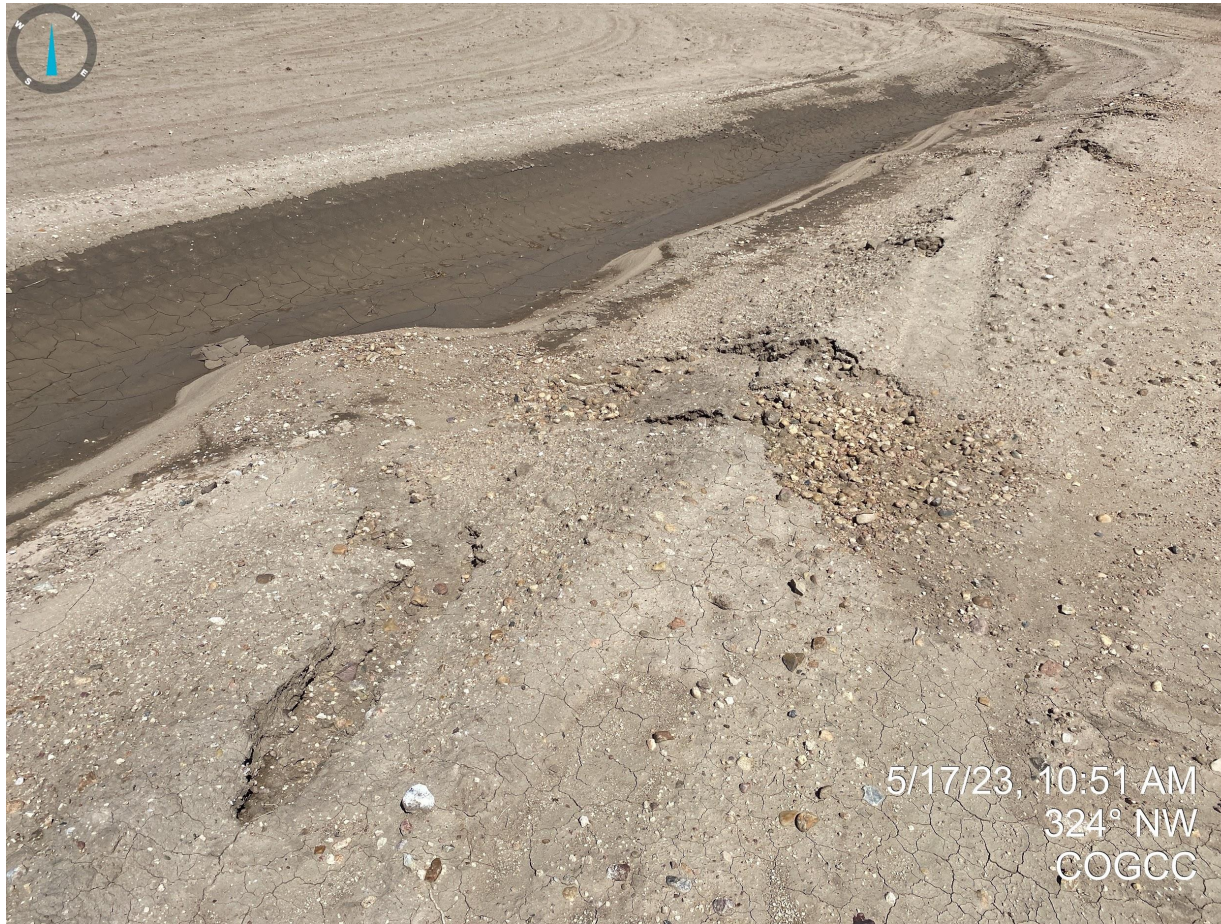
Photo 9. From the western portion of the production area. Portions of the production area do not appear stabilized with evidence of rill erosion and sediment deposition in the stormwater ditches. Additional stormwater BMP maintenance will need to be performed.
