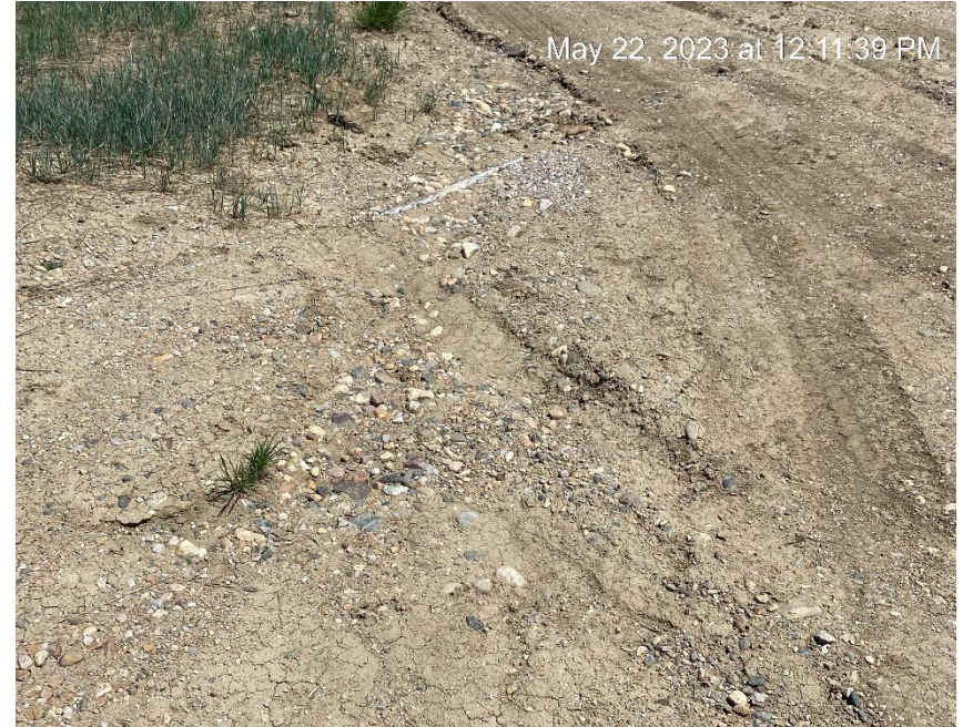
Location erosion at access road entrance
