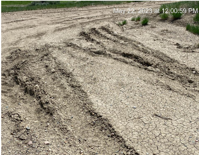
Lack of stabilization and sediment migration
