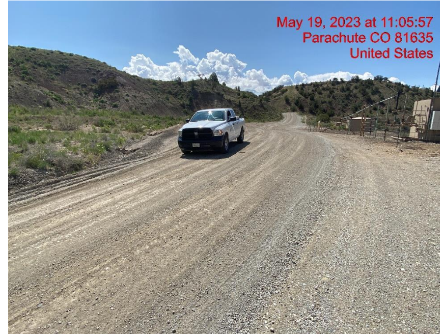
Insufficient Vehicle Tracking BMPs at Location Entrance/Exit – Photo #03654
