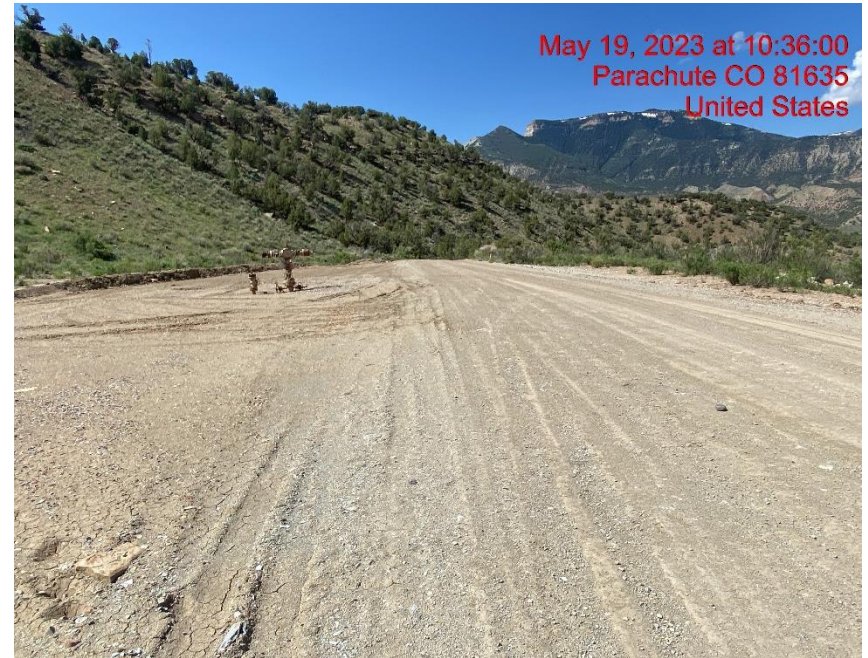
Insufficient Vehicle Tracking BMPs at Location Entrance/Exit – Photo #03608
