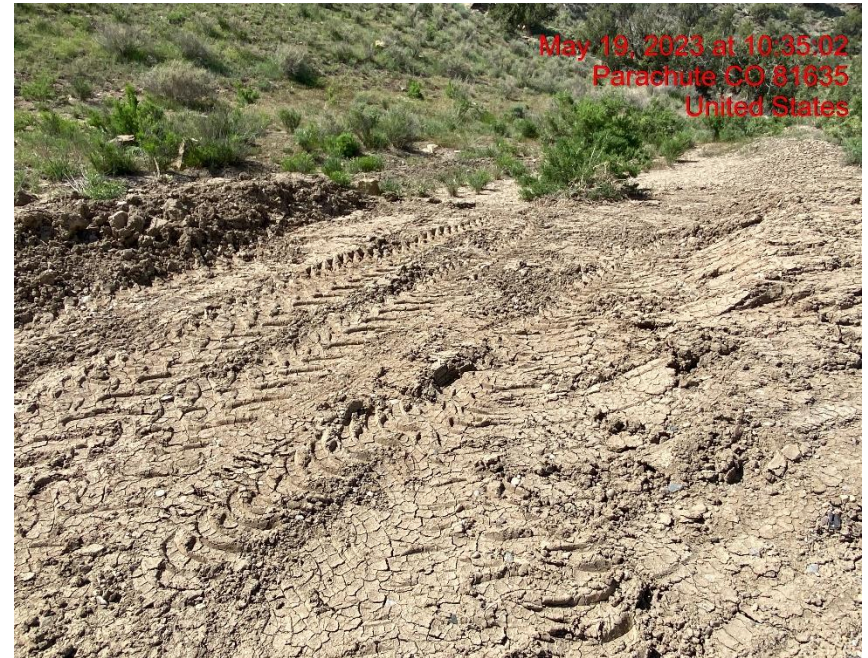
Lack of Stabilization/Degradation Causing Transportation of Sediment – Photo #03604
