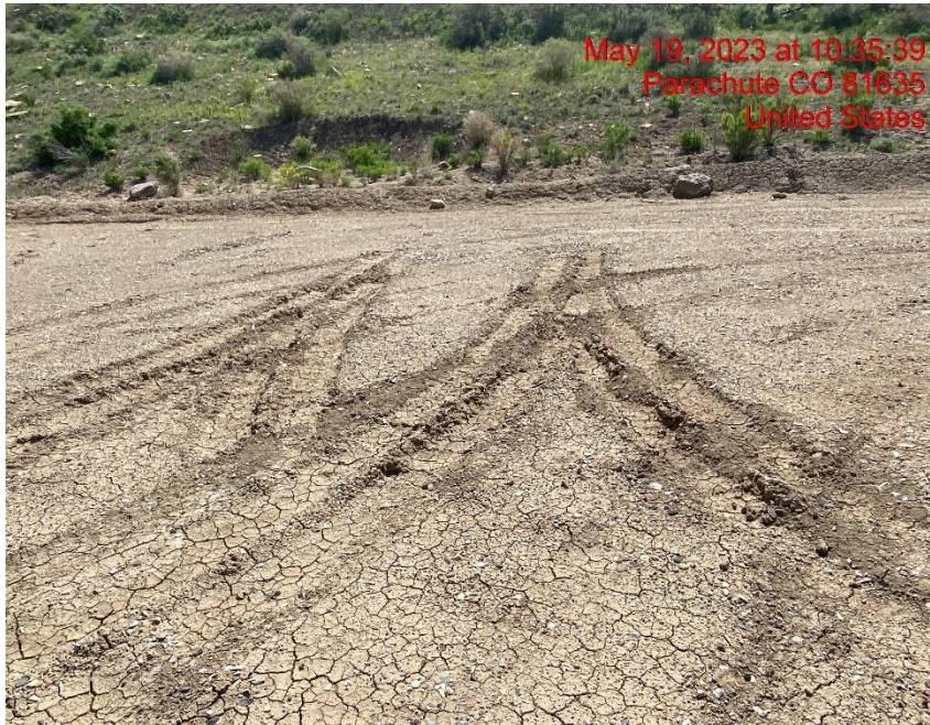
Location Lacks Stabilization – Photo #03607
