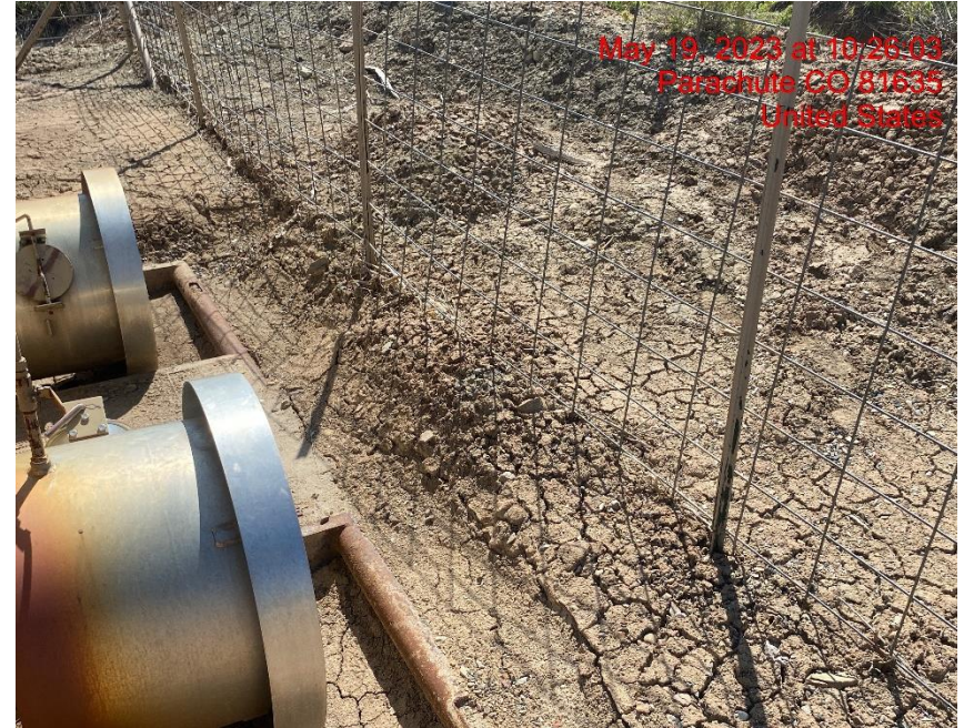
Sediment Encroaching on Equipment – Photo #03590
