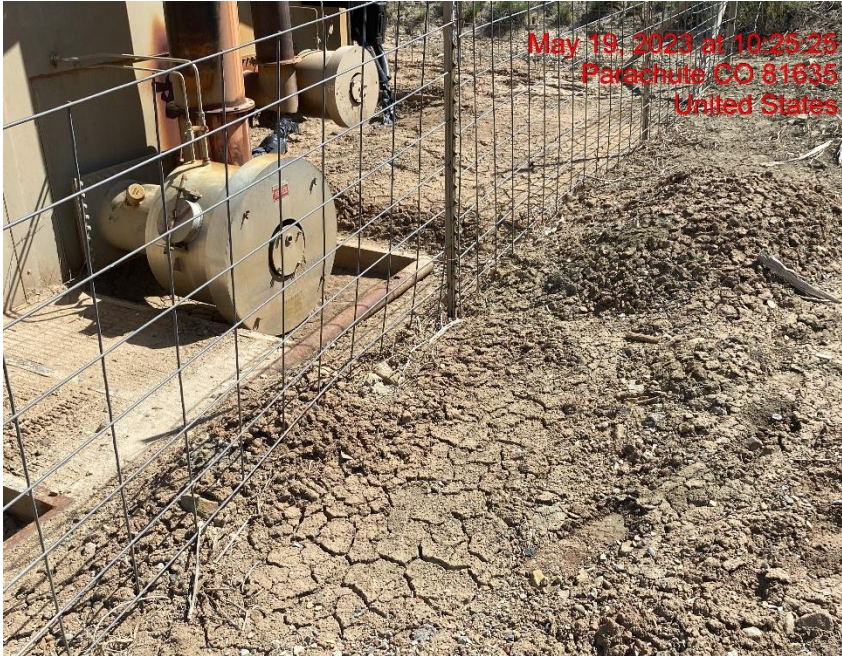
Sediment Encroaching on Equipment – Photo #03589
