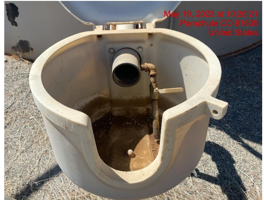
Open-Ended Load Line – Photo #03591
