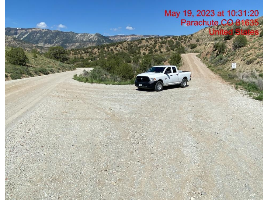
Insufficient Vehicle Tracking BMPs at Location Entrance/Exit – Photo #03598
