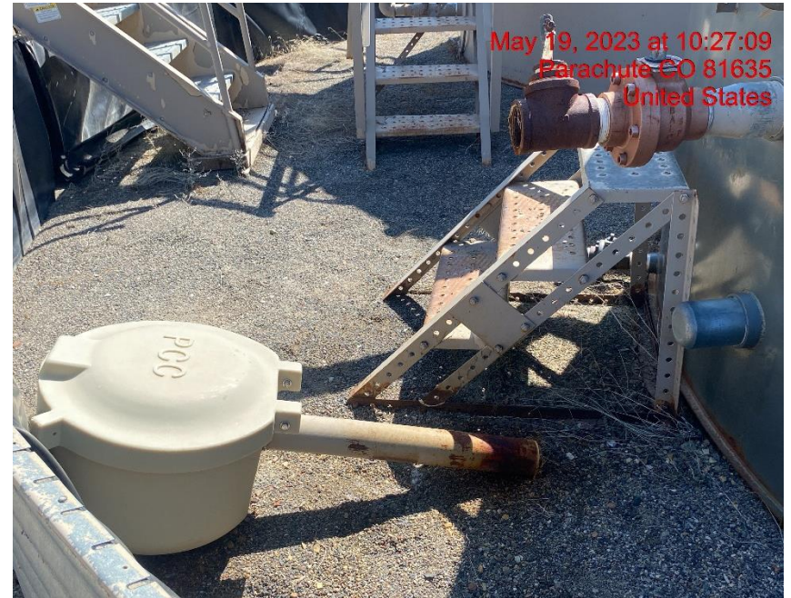
Unsecured Load Line – Photo #03593
