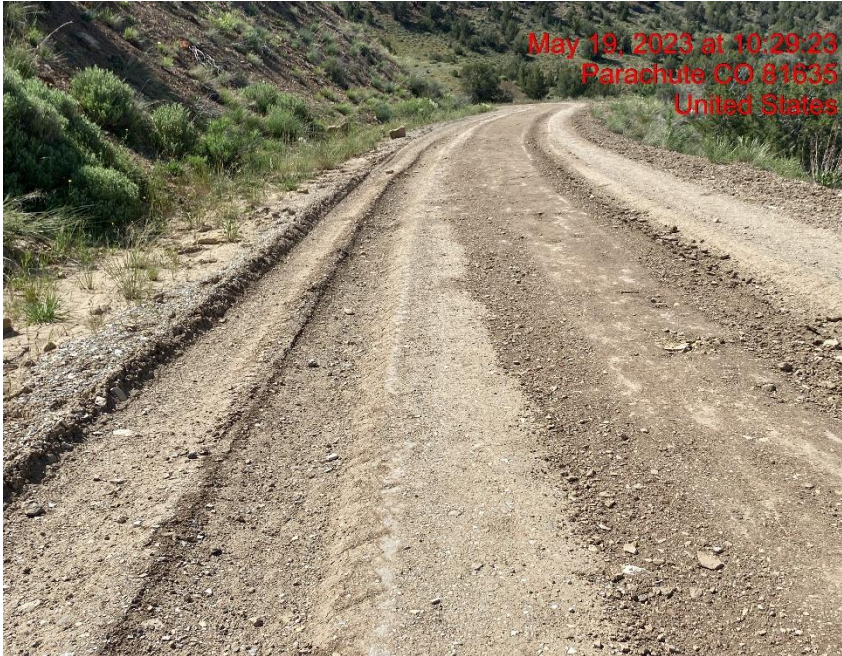
Lease Road Lacks Stabilization – Photo #03595
