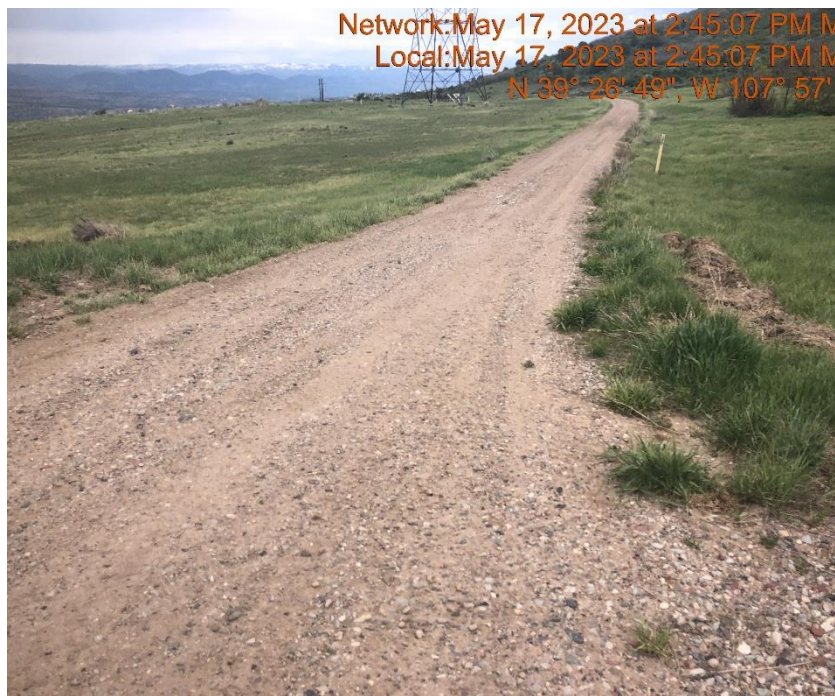
Photo #42 Insufficient tracking BMP at entrance to location to minimize the transport of sediment.
