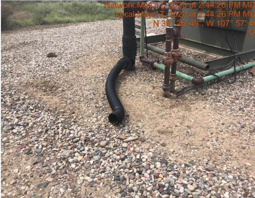
Photo #39 Flowline heating insulation open ended.
