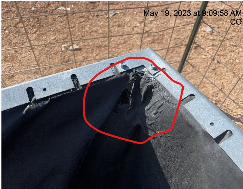
Photo # 8179 Containment liner needs maintenance
