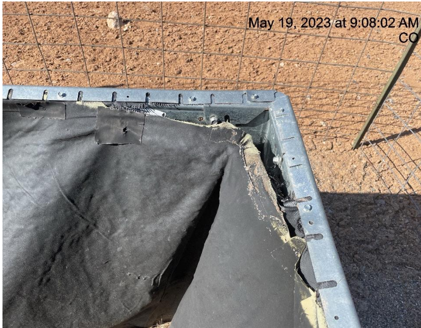
Photo # 8173 Containment liner needs maintenance
