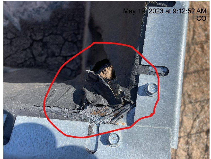
Photo # 8180 Containment liner needs maintenance
