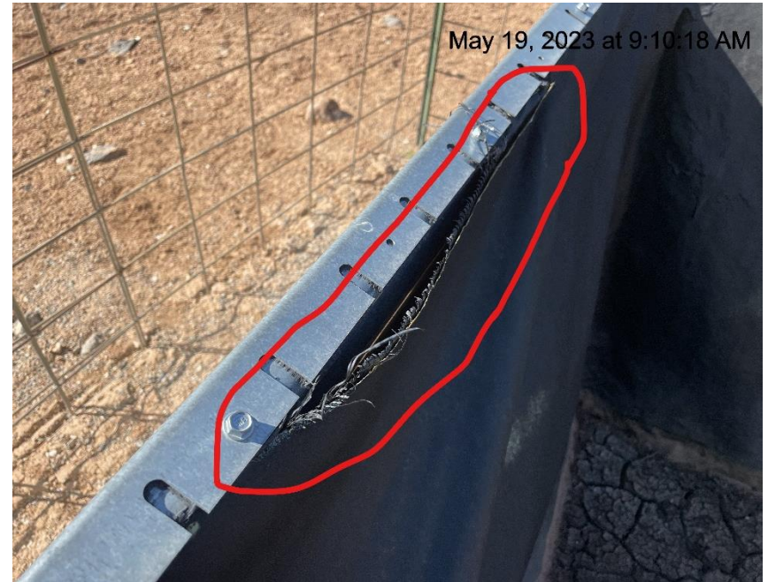
Photo # 8178 Containment liner needs maintenance
