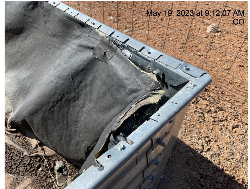
Photo # 8174 Containment liner needs maintenance
