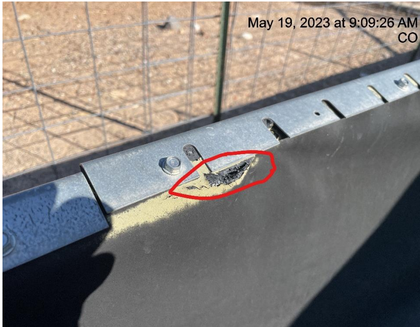
Photo # 8177 Containment liner needs maintenance
