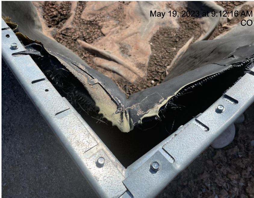
Photo # 8181 Containment liner needs maintenance
