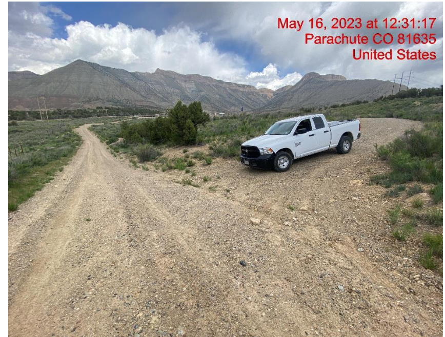
Insufficient Vehicle Tracking BMPs at Location Entrance/Exit – Photo #03574
