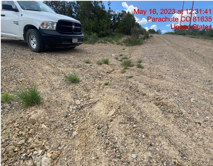
Rill Erosion Transporting Sediment Across Access Road – Photo #03575
