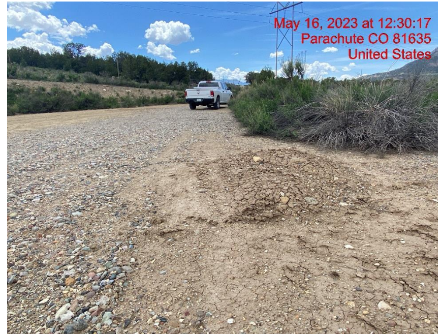
Unprotected Soil Stockpile – Photo #03571
