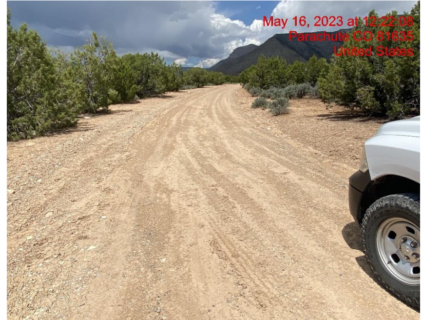
Insufficient Vehicle Tracking BMPs at Location Entrance/Exit – Photo #03559
