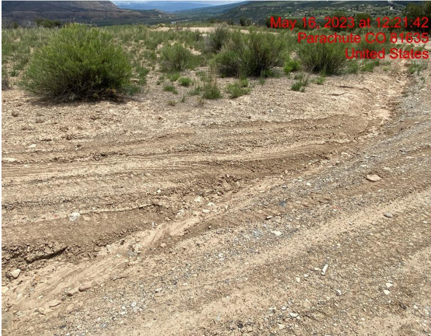
Rill Erosion Transporting Sediment Across Lease Road – Photo #03558
