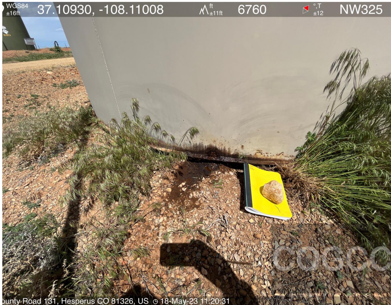
Photo #3. View of inadequate tank integrity, leak.
