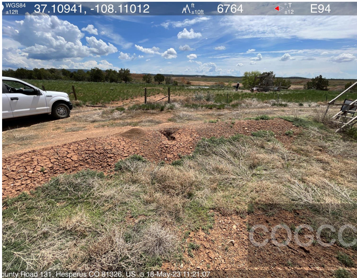
Photo #1. Overview of well location, animal burrow in tank berm.
