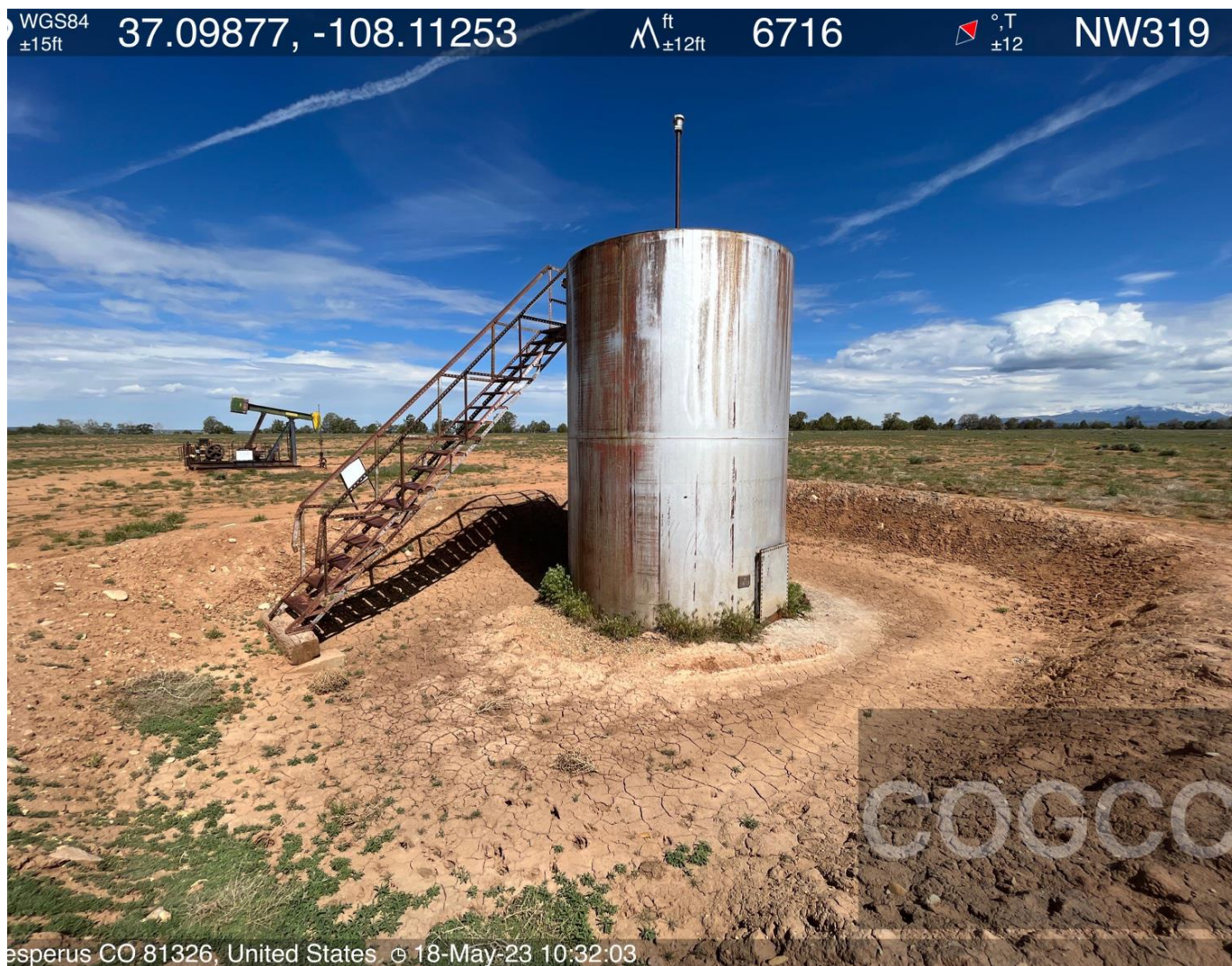
Photo #3. View of crude oil tank and containment berm.
