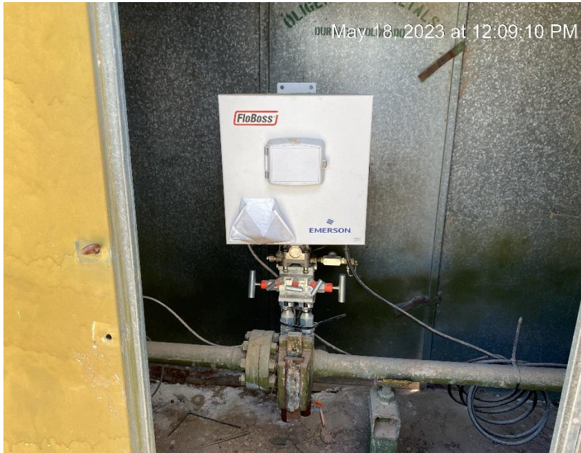
Gas meter calibration not visibly displayed
