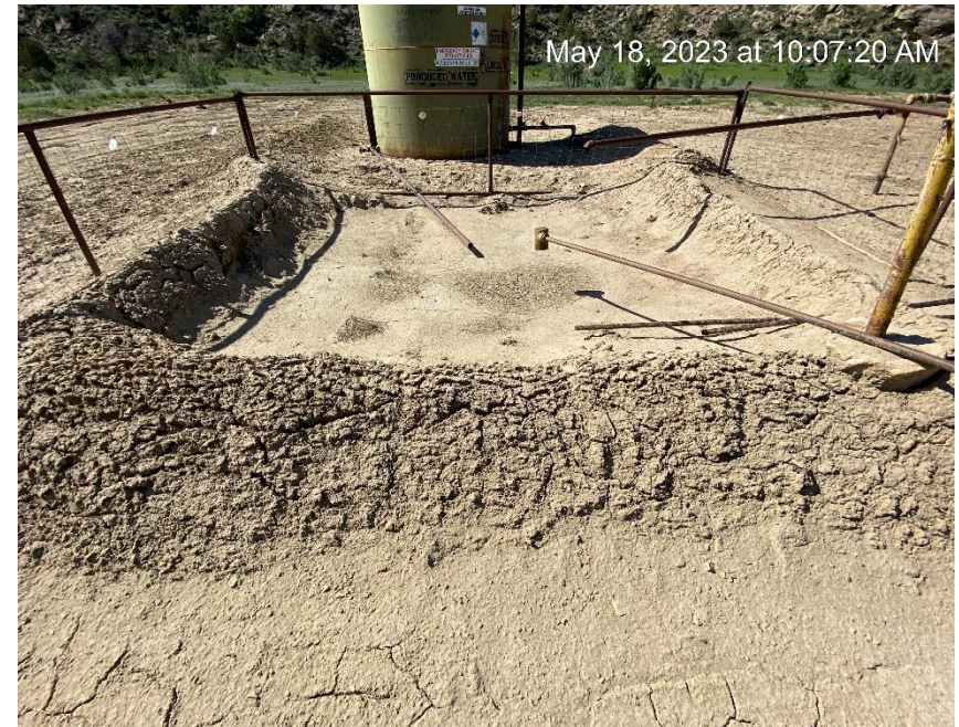
Water tank and production pit berms
