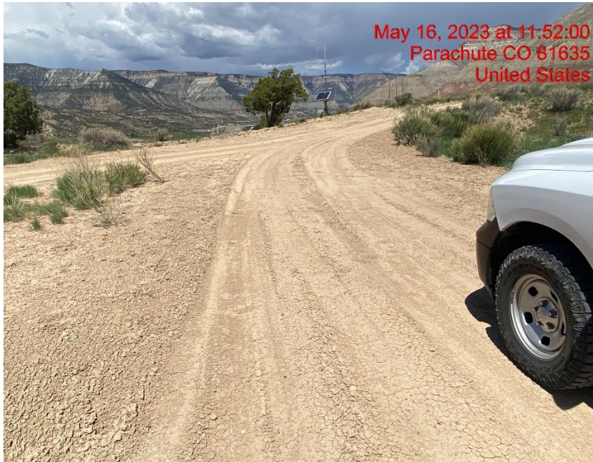
Insufficient Vehicle Tracking BMPs at Location Entrance/Exit – Photo #03492
