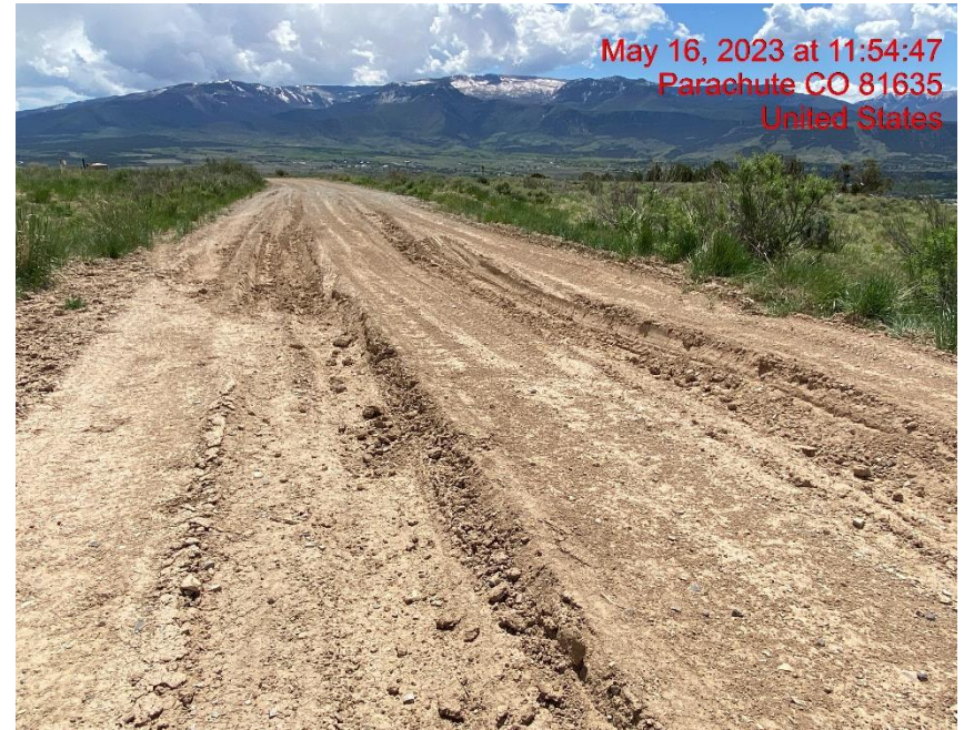
Access Road Lacks Stabilization – Photo #03496
