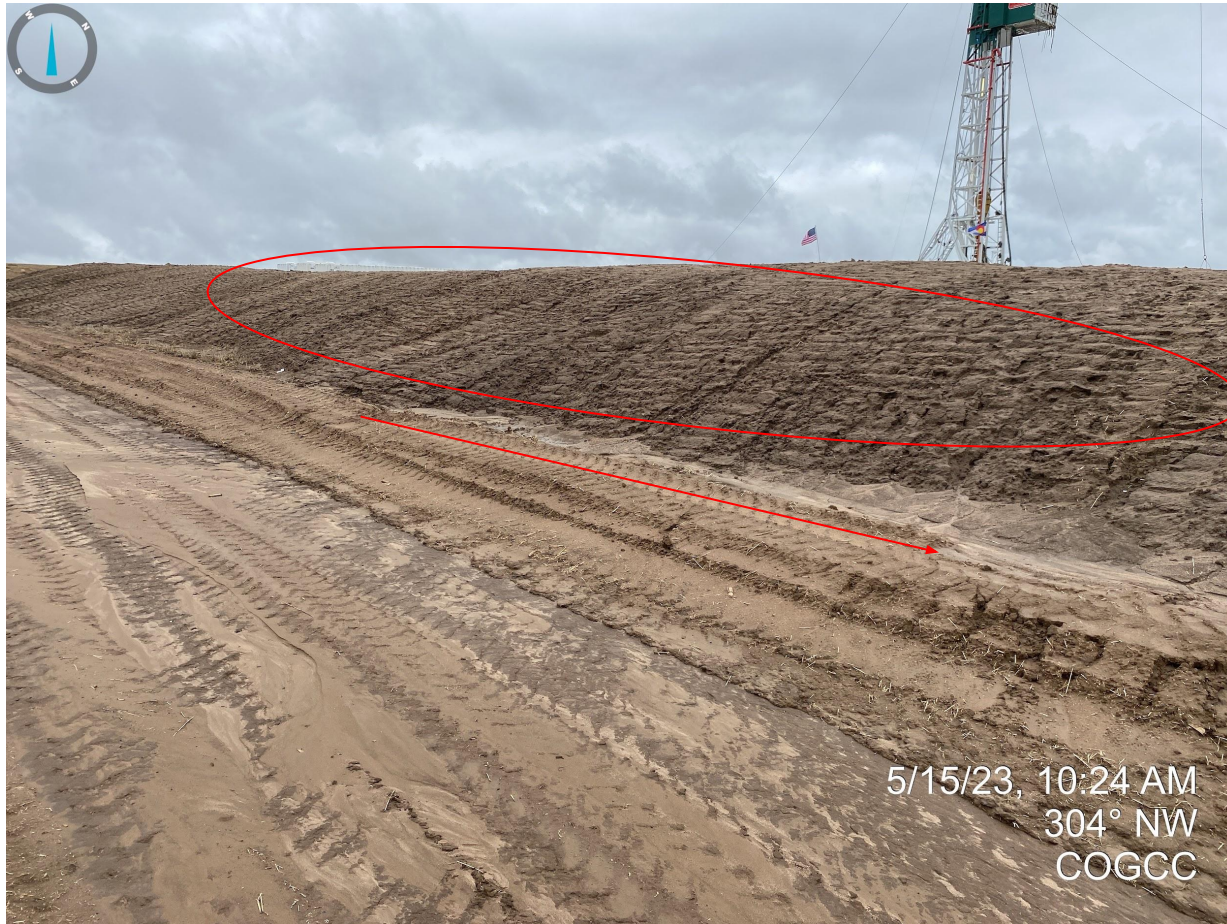
Photo 9. Taken from the eastern end of the stockpile. See comments in Photo 8. Circle identifying rill erosion and arrow illustrating sediment deposition.
