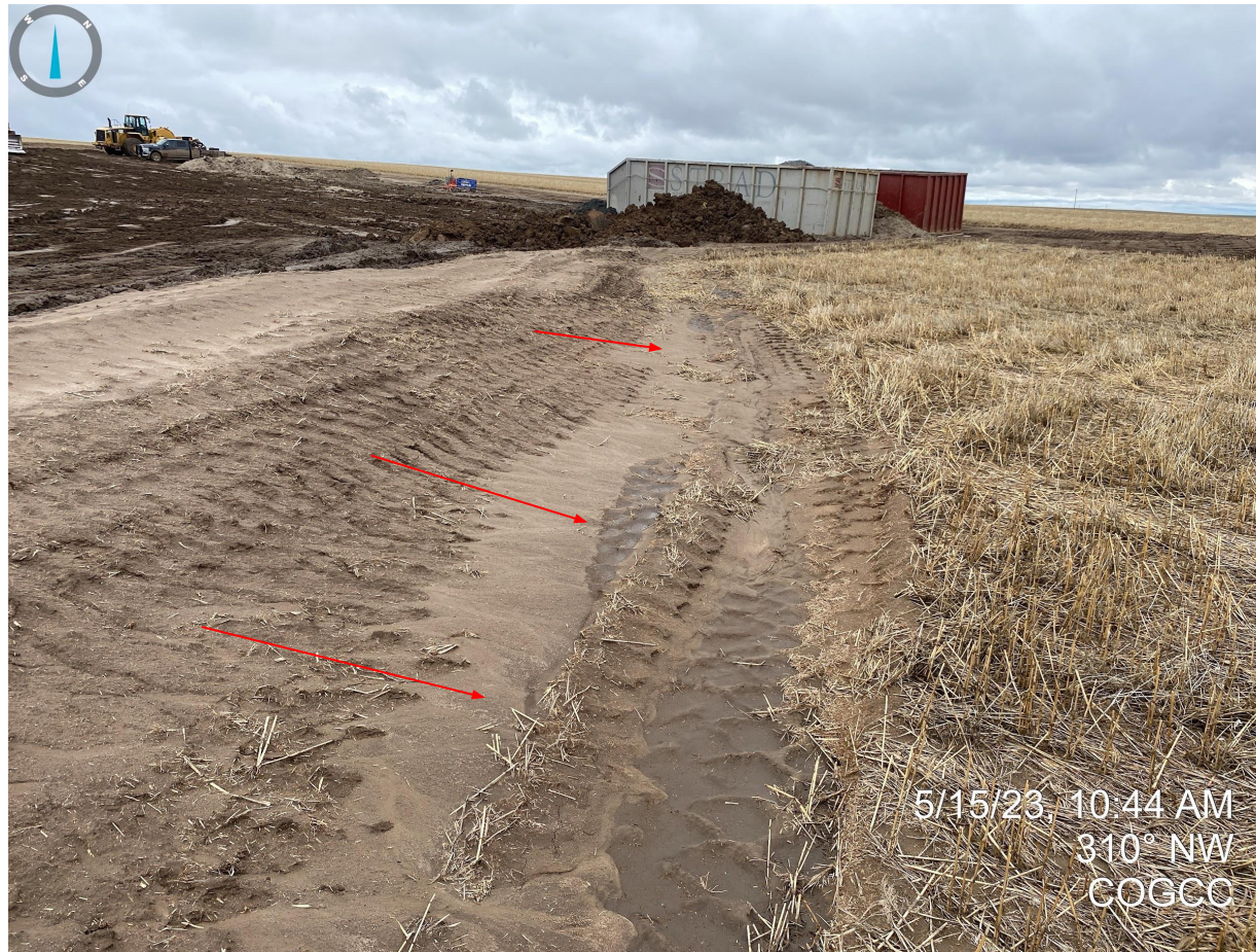
Photo 23. Taken from the eastern portion of the location, near the entrance. Berm material does not appear to be properly stabilized with evidence of sediment deposition.
