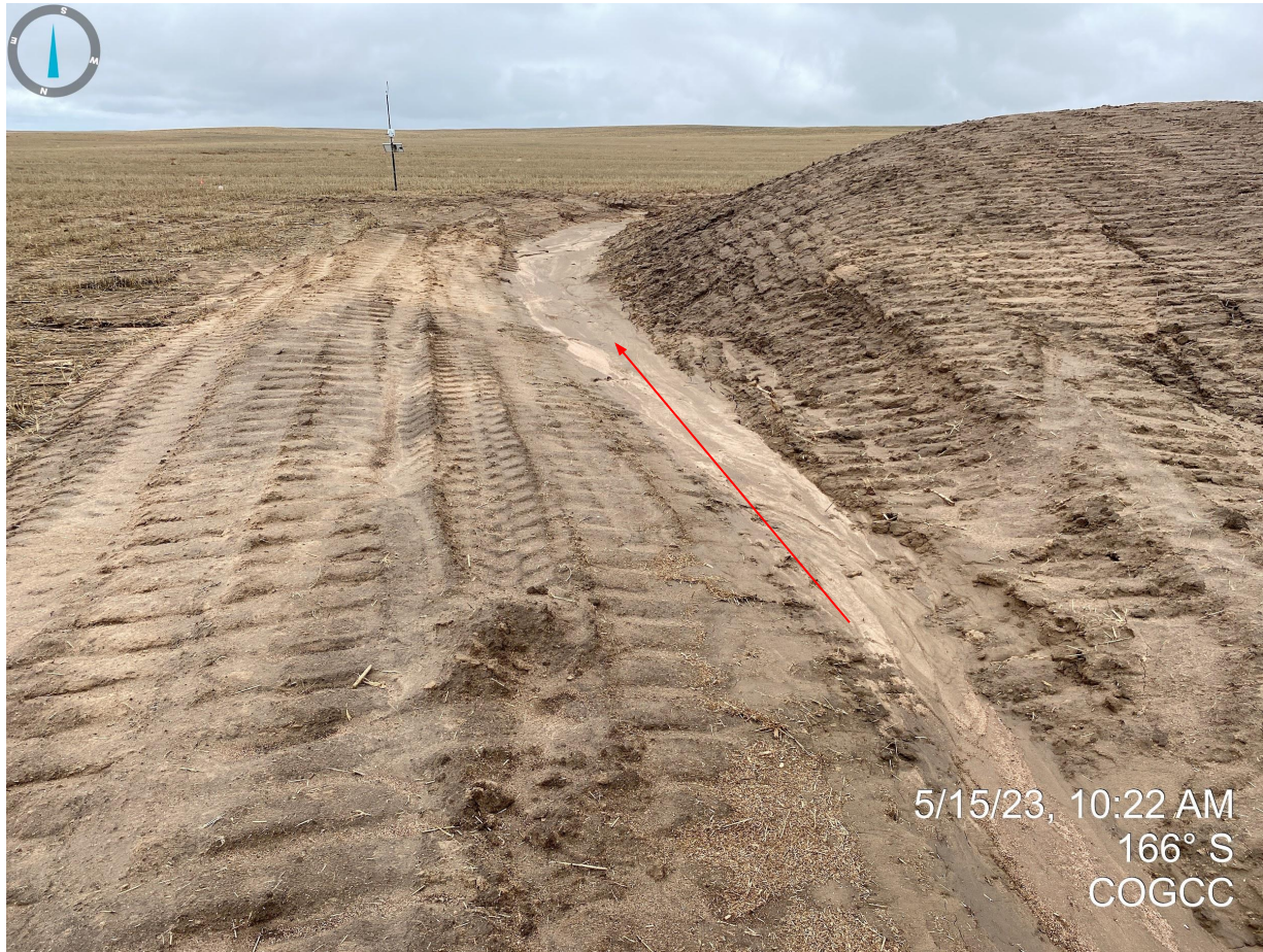
Photo 5. Ditch on the east side of the location appears to be filled with sediment; advise ditch maintenance in order to handle/control future stormwater events.
