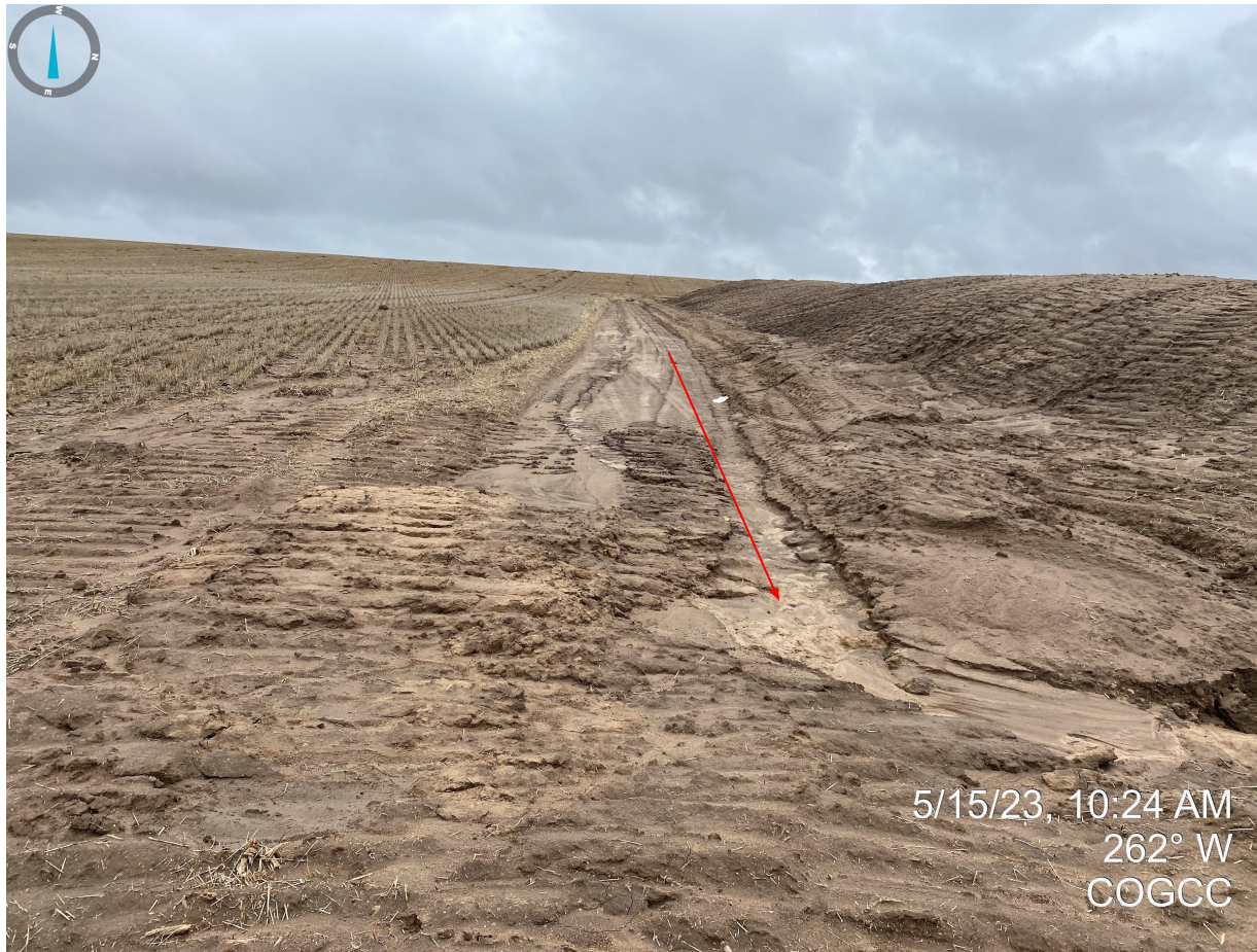
Photo 11. Facing west on the southern edge of the location. Photo illustrates rill erosion occurring on areas grubbed, with no apparent stormwater BMPs observed. More robust stormwater BMPs will need to be implemented to control stormwater run-on and run-off, and prevent further site degradation.
