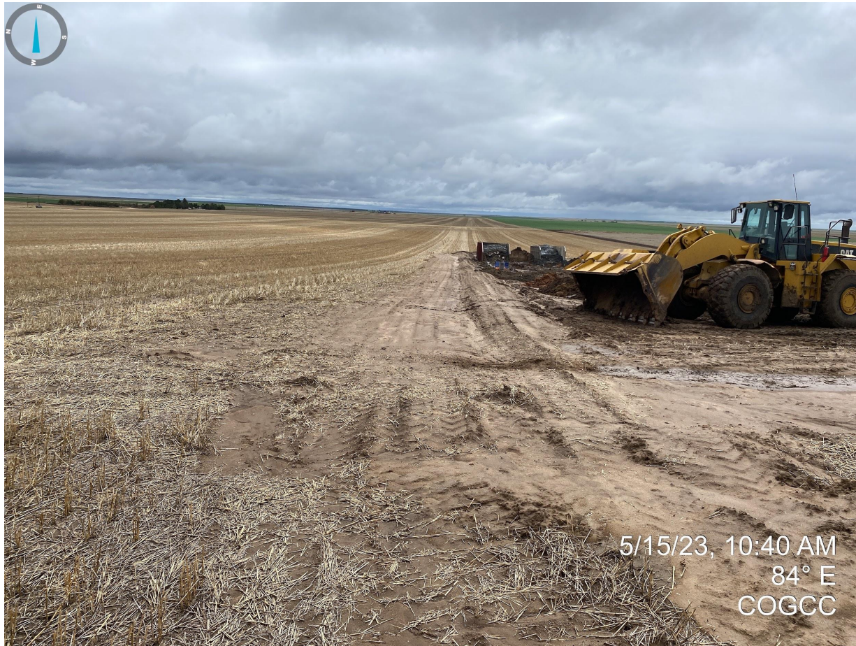
Photo 19. Facing east from the northwest corner of the location. Photo illustrates that stormwater BMPs appear to be inadequate for this location. Grubbed areas have no apparent stormwater/erosion controls to prevent sediment transport.
