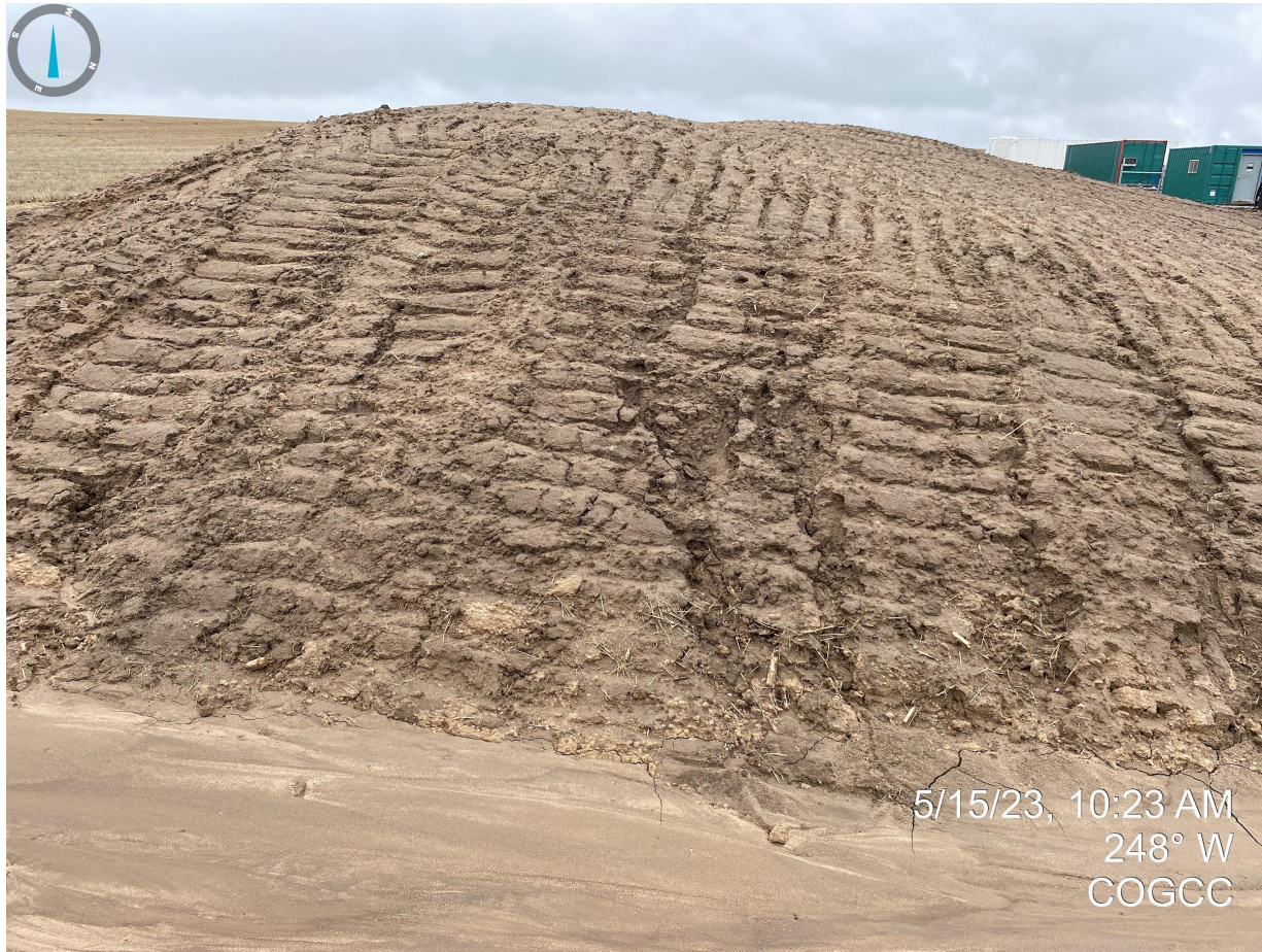
Photo 8. Facing west at the east end of the topsoil stockpile. Rill erosion evident on the walls of the stockpile. While equipment tracking appears to have been performed previously, additional short term stabilization work will need to be performed to prevent further erosion from occurring.
