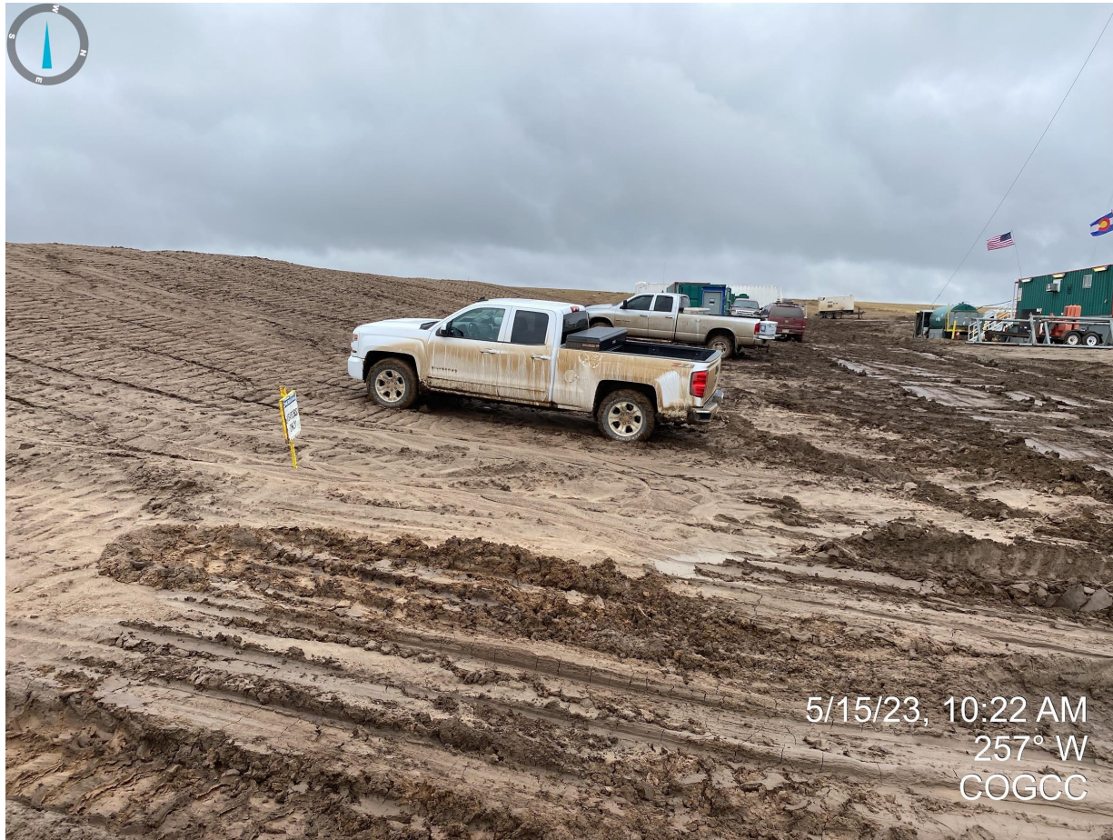
Photo 3. Facing west at topsoil stockpile. Vehicles and equipment were observed to be parked on the topsoil stockpile.
