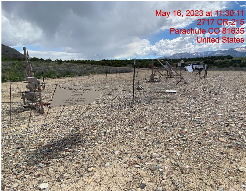
Wellhead Fencing Not Serviceable – Photo #03448
