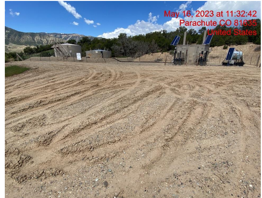
Location Lacks Stabilization – Photo #03453
