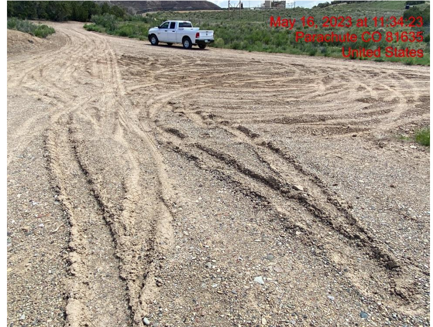
Location Lacks Stabilization – Photo #03460
