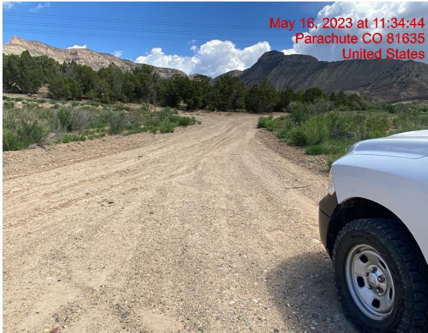
Insufficient Vehicle Tracking BMPs at Location Entrance/Exit – Photo #03461
