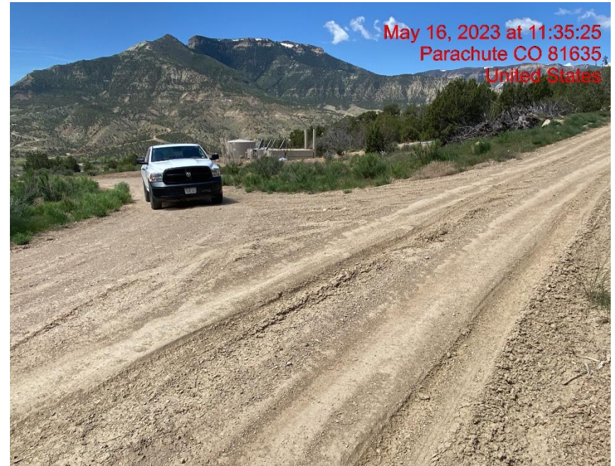
Insufficient Vehicle Tracking BMPs at Location Entrance/Exit – Photo #03462
