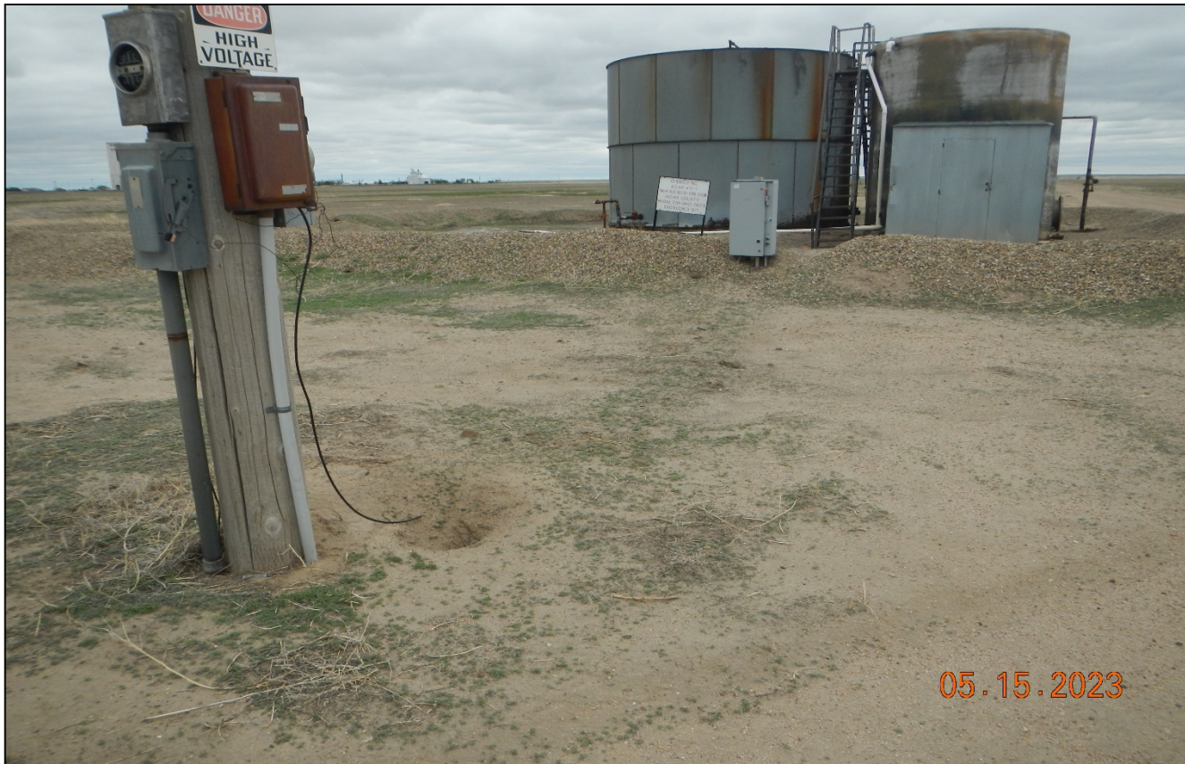
Photo 5. The electric line appears to have been buried to the tank battery. The line still hang by the pole and should be better protected with pipe, ect.
