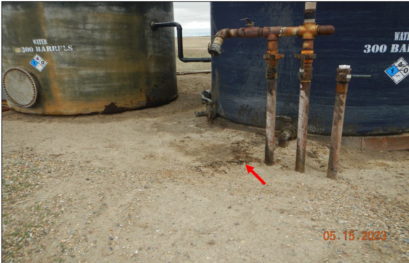
Photo 2. There is still oil stained soil around the tank from a spill contained inside the bermed area.
