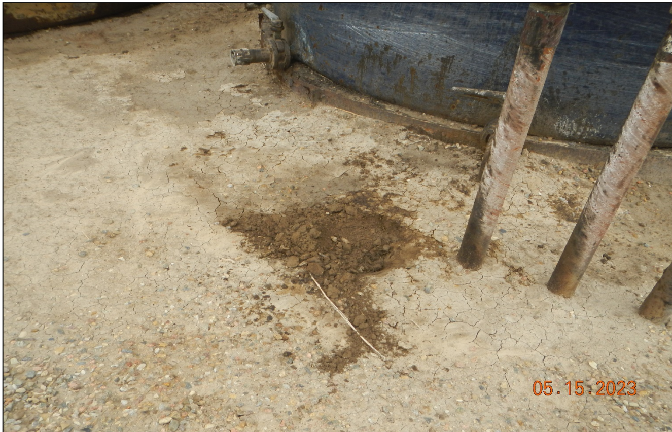
Photo 3. There is still oil stained soil around the tank from a spill contained inside the bermed area.
