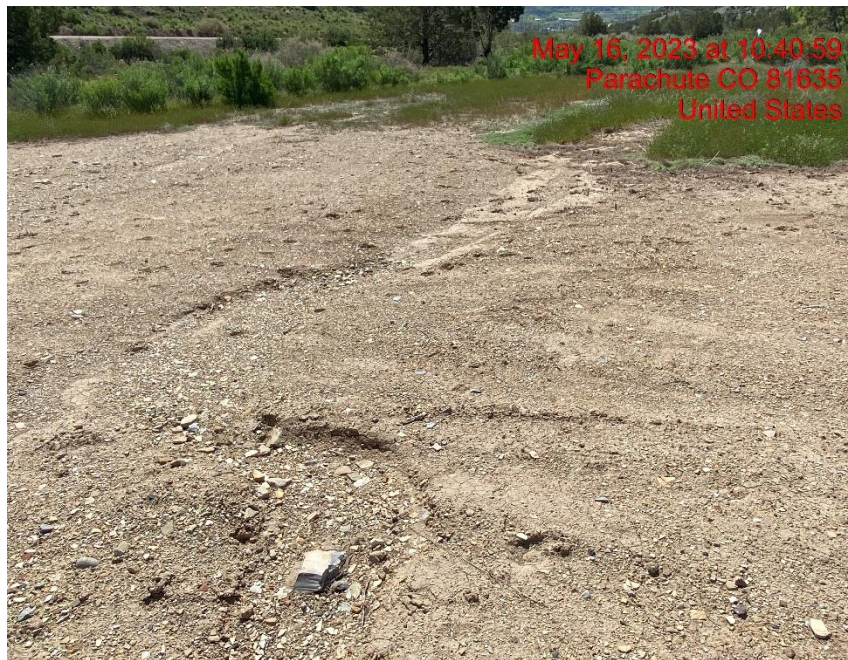
Rill Erosion Transporting Sediment Off-Location – Photo #03372
