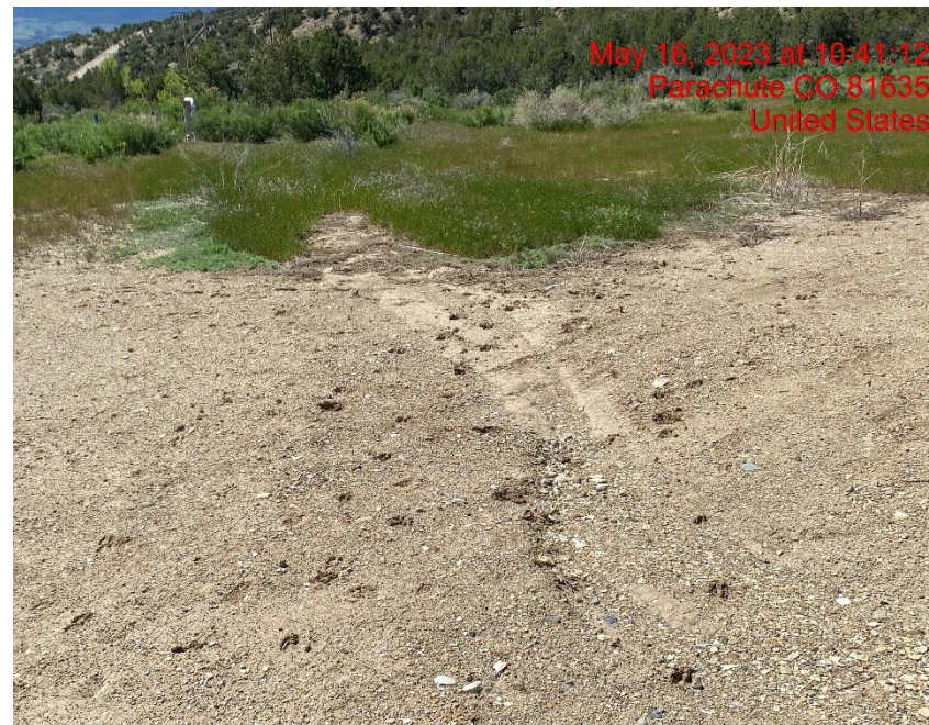
Rill Erosion Transporting Sediment Off-Location – Photo #03374
