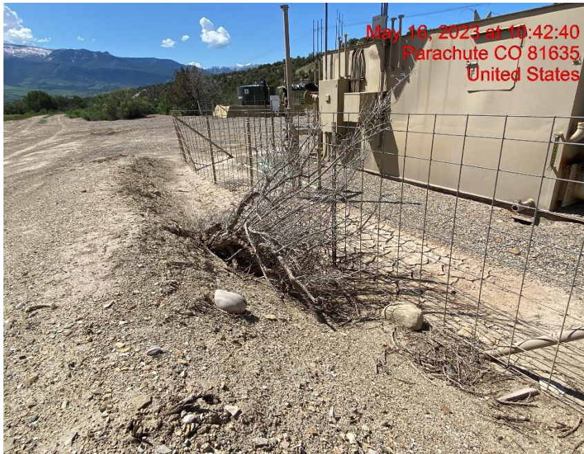
Site Degradation from Plow Causing Sediment Transportation and Lack of Stabilization – Photo #03376
