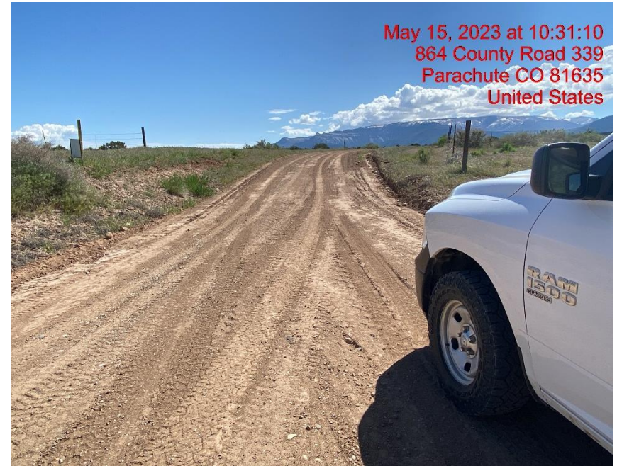
Insufficient Vehicle Tracking BMPs at Location Entrance/Exit – Photo #03343
