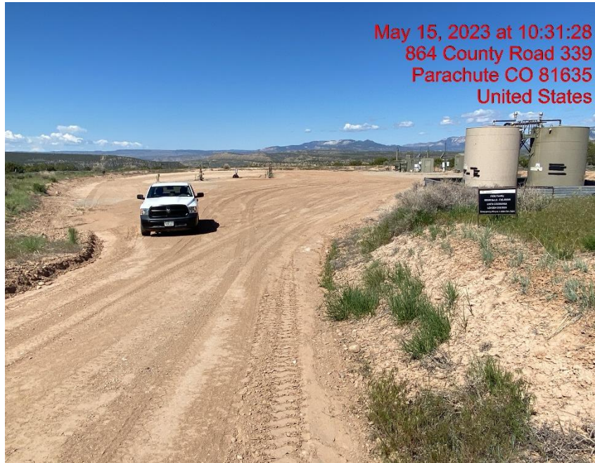
Insufficient Vehicle Tracking BMPs at Location Entrance/Exit – Photo #03344
