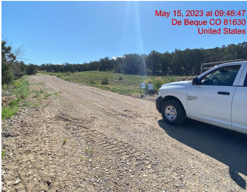
Insufficient Vehicle Tracking BMPs at Location Entrance/Exit – Photo #03293
