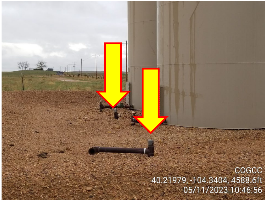
Photo 3 – Unmarked Risers
