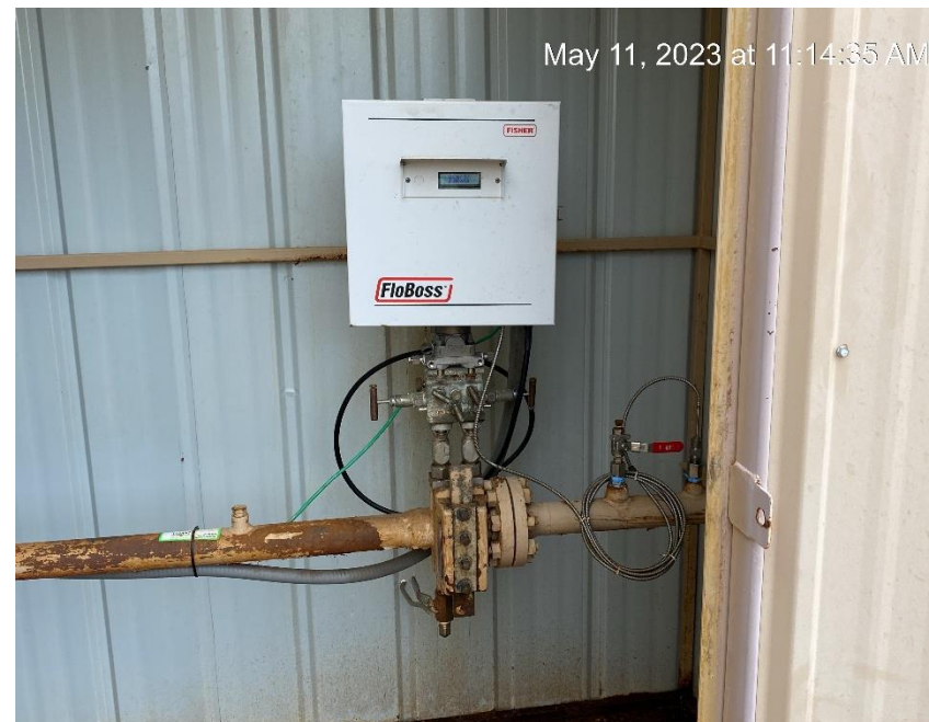
Gas meter calibration not visibly displayed
