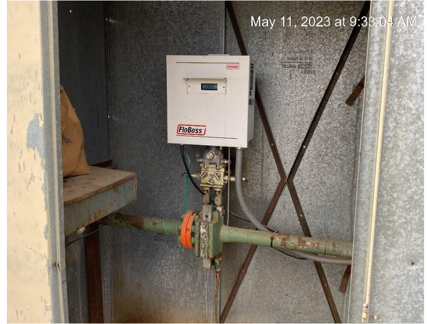
No visible display of gas meter calibration
