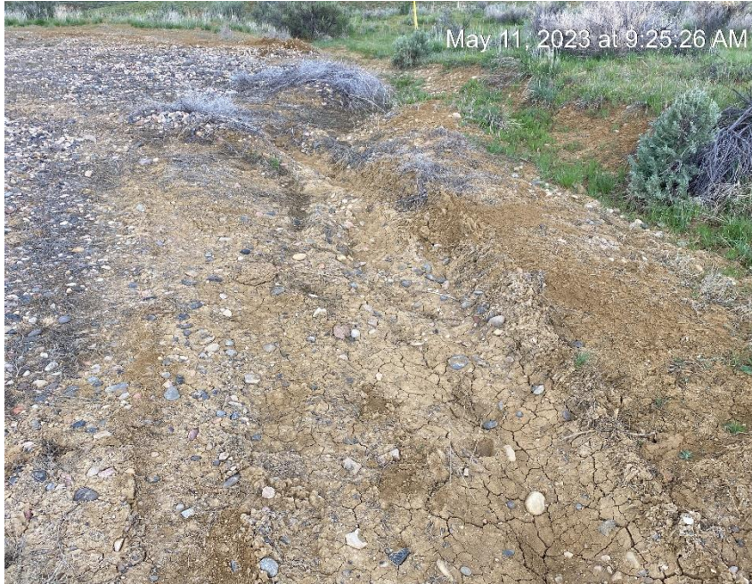
Diversion ditch and berm damage
