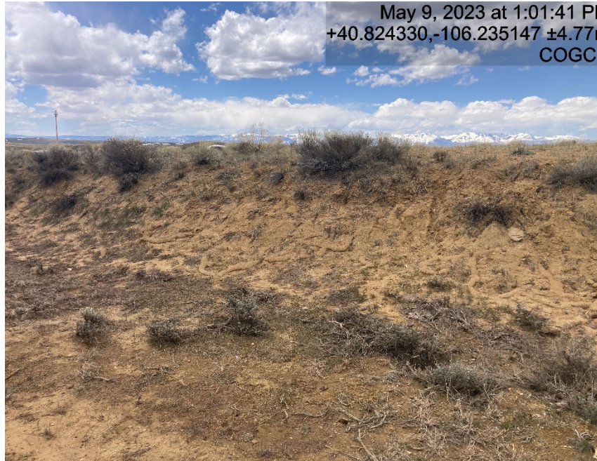
Cut slope shows signs of lack of stabilization
