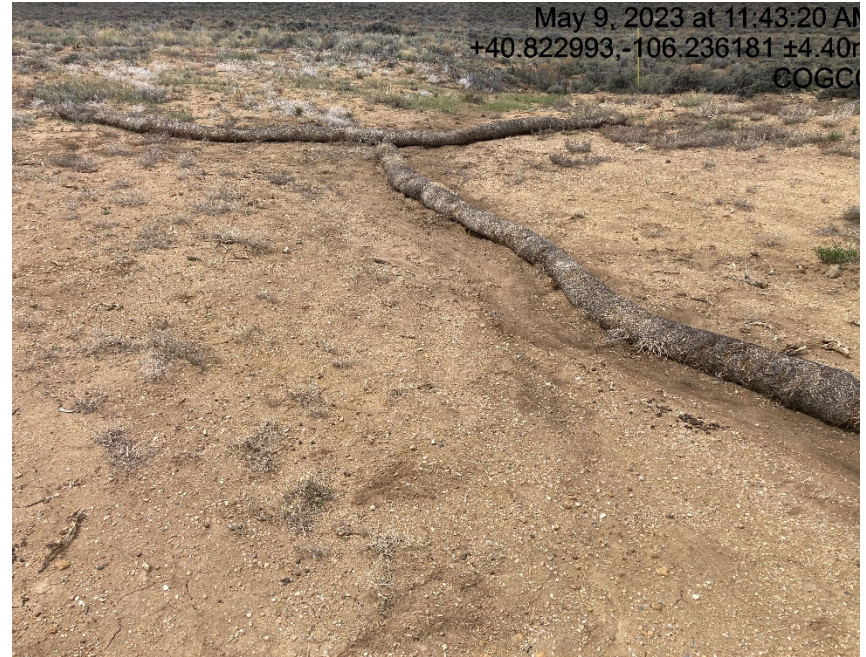
Improperly installed BMP's
