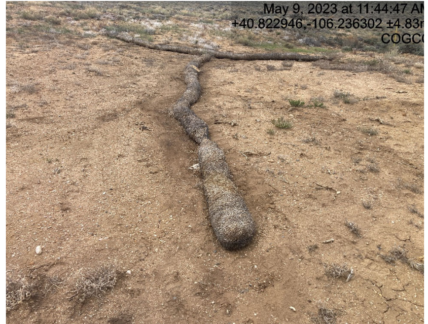
Improperly installed BMP's
