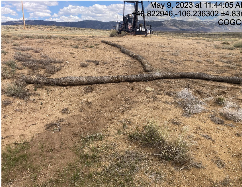
Improperly installed BMP's
