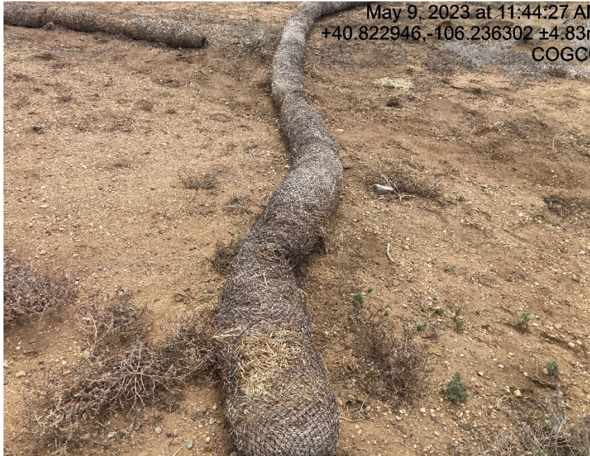
Improperly installed BMP's
