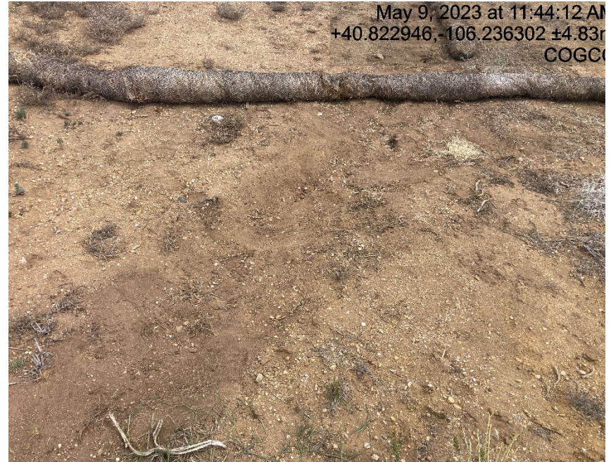
Improperly installed BMP's
