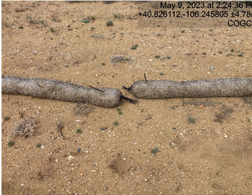
Improperly installed BMP's
