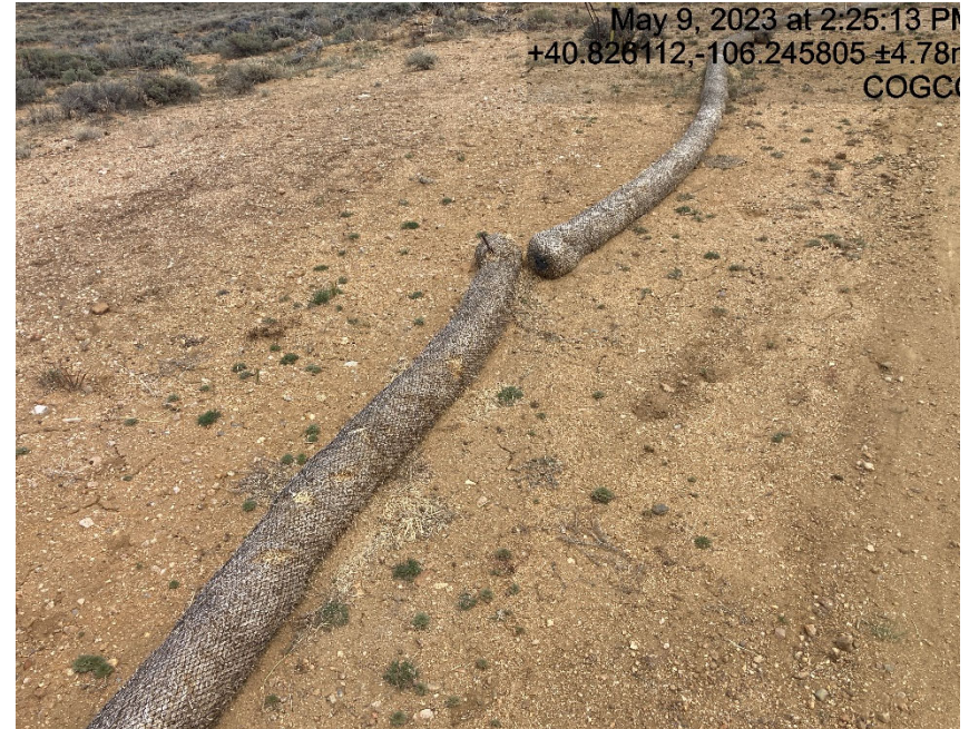
Improperly installed BMP's
