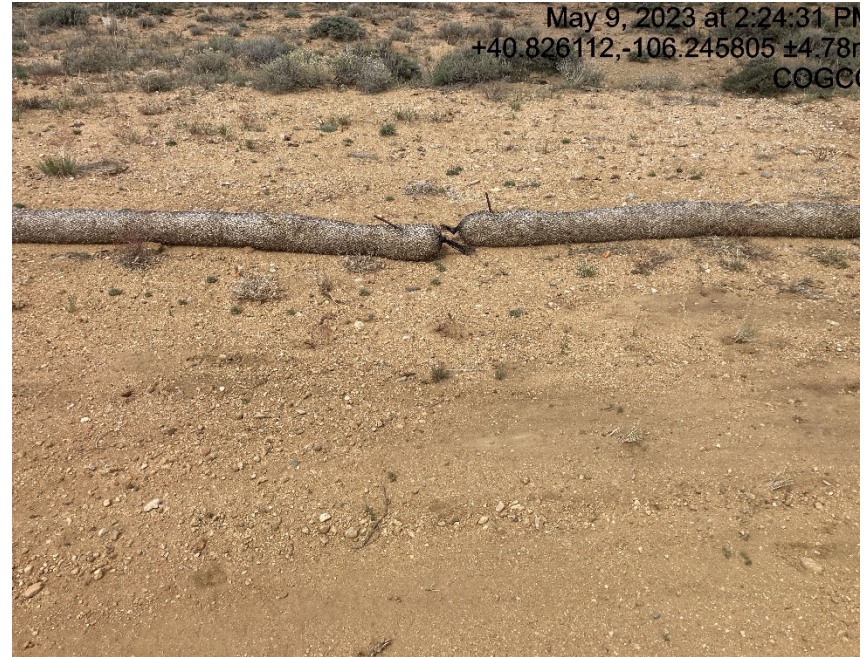
Improperly installed BMP's
