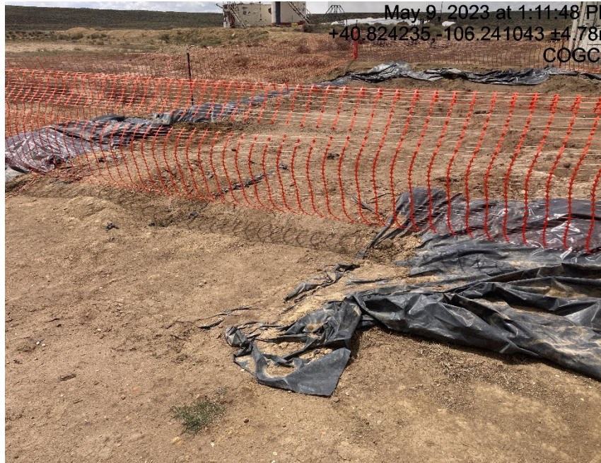
Contaminated soil migrating out of containment
