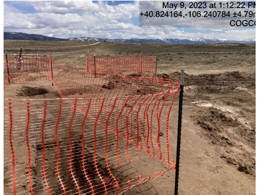
Excavated area of contaminated soil
