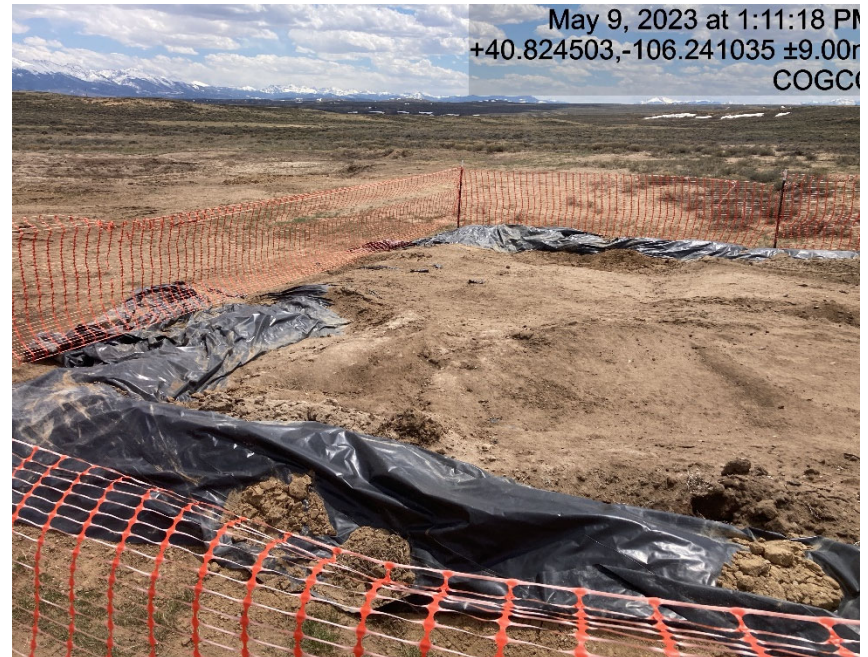
Contaminated soil migrating out of containment
