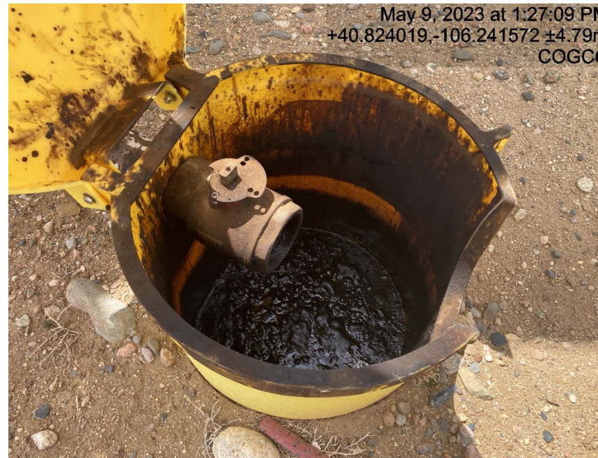
Valve on tank missing cap/plug
