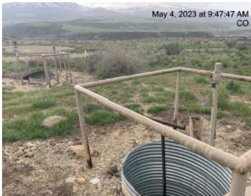
Photo # 6922 From Inspection 708900405 conducted on 05/04/2023 Open cellar/wildlife hazard (Cellar is just off lease road approximately 25-50 yards past CLOUGH 2A pad)
