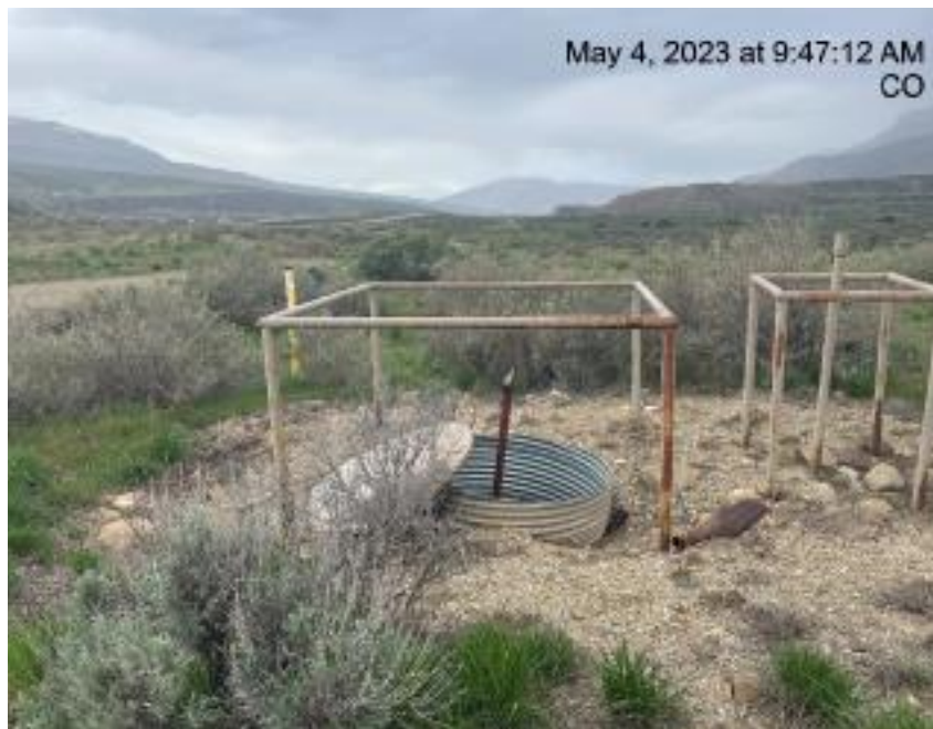
Photo # 6921 From Inspection 708900405 conducted on 05/04/2023 Open cellar/wildlife hazard (Cellar is just off lease road approximately 25-50 yards past CLOUGH 2A pad)
