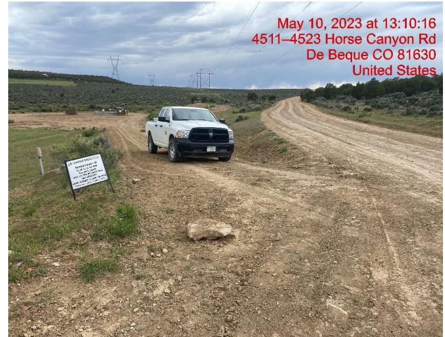
Insufficient Vehicle Tracking BMPs at Location Entrance/Exit – Photo #03175
