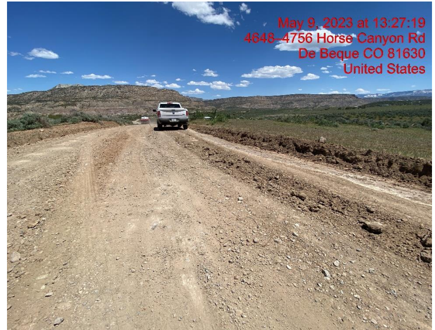
Lease Road Degradation/Transport of Sediment – Photo #03149
