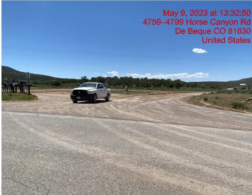
Insufficient Vehicle Tracking BMPs at Lease Road Entrance/Exit – Photo #03158
