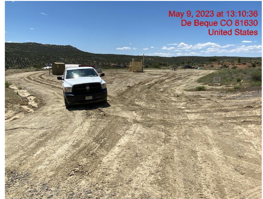
Insufficient Vehicle Tracking BMPs at Location Entrance/Exit – Photo #03146
