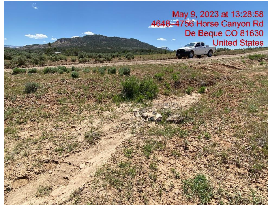
Insufficient Check Dam BMP – Photo #03153
