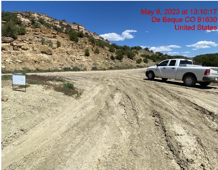
Insufficient Vehicle Tracking BMPs at Location Entrance/Exit – Photo #03145
