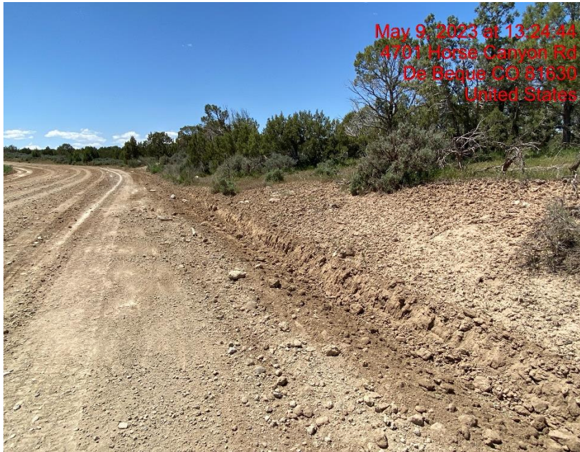
Lease Road Degradation/Transport of Sediment – Photo #03148
