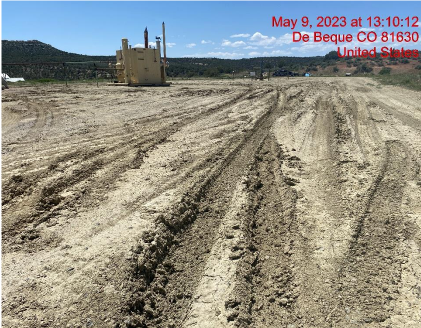
Location Lacks Stabilization – Photo #03144
