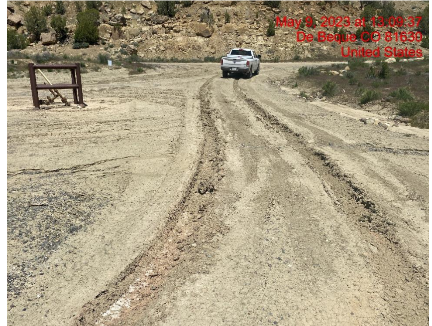
Location Lacks Stabilization – Photo #03141
