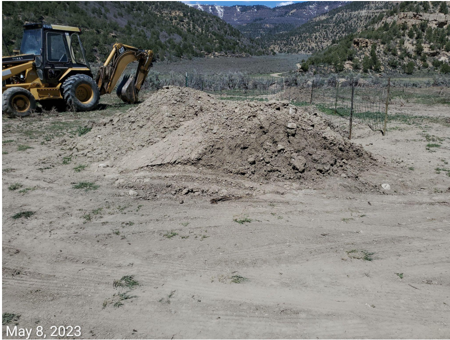
Photo 2: BMPs missing from stockpiled soils on the Location.
