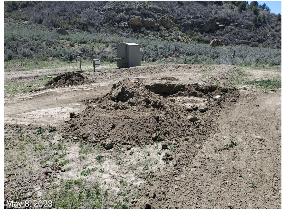
Photo 2: BMPs missing from stockpiled soils on the Location.
