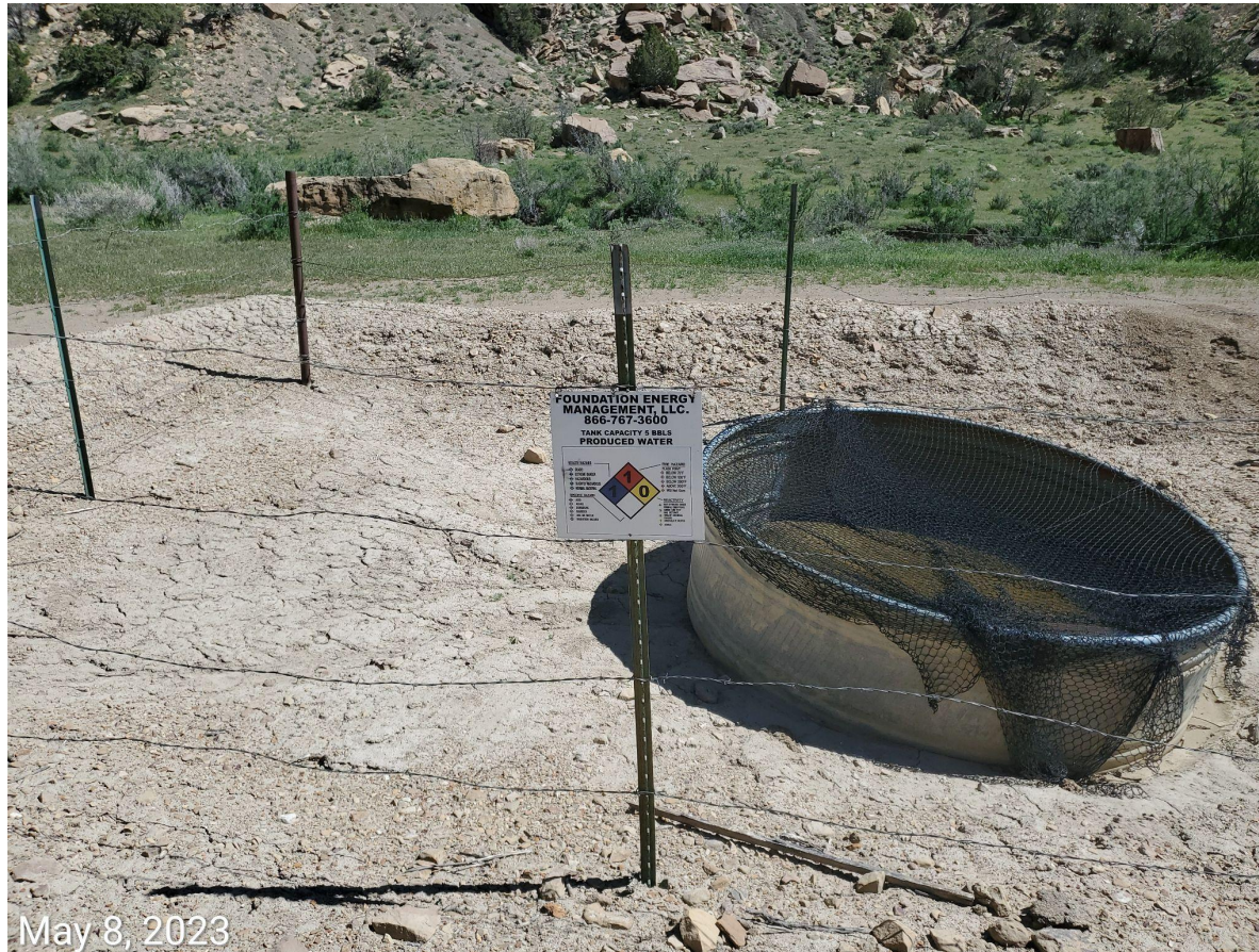
Photo 6: Photo of the produced water tank. Photo shows signage/labeling at the tank remains out of compliance with Rule 605 requirements.
