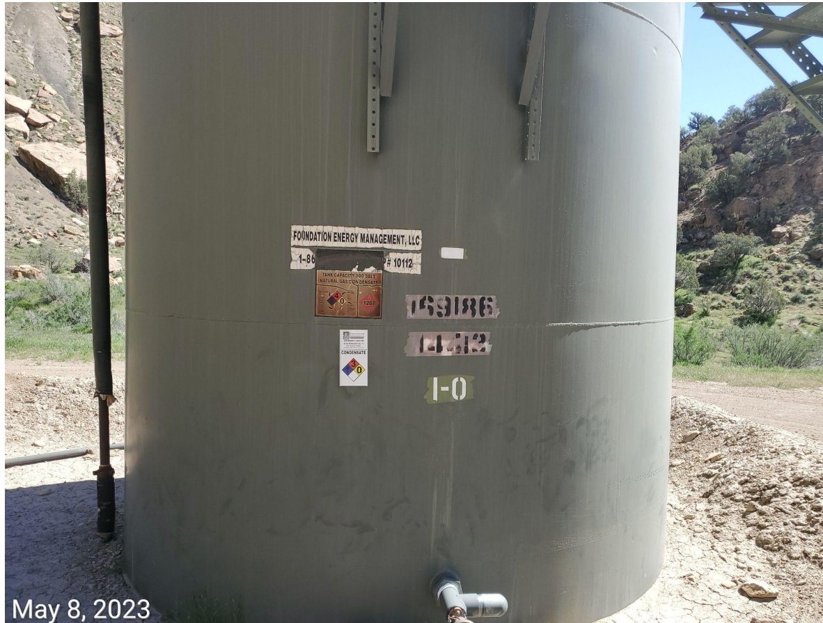
Photo 5: Photo of the condensate tank. Photo shows signage/labeling at the tank remains out of compliance with Rule 605 requirements.
