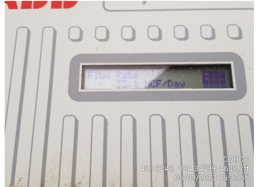
Photo 2 – Appears to have Gas Flowing through Sales Meter
