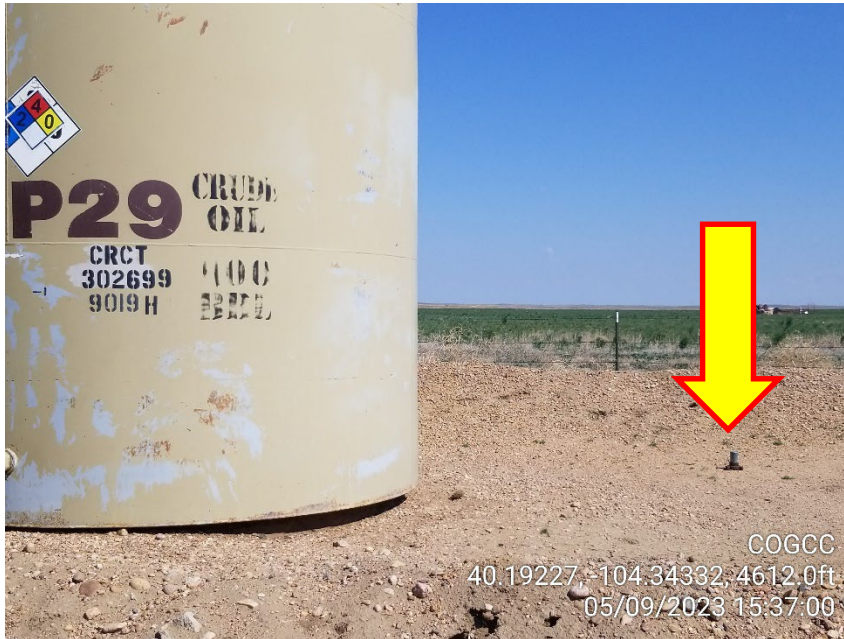
Photo 9 – Unmarked Risers in Tank Berm
