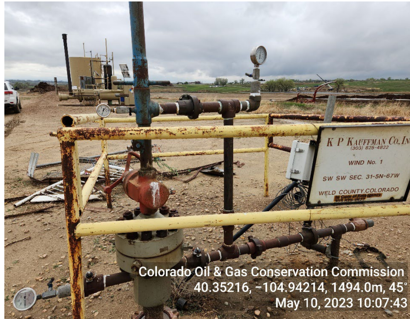
Photo 9: Valves appear to be open, pressure present on gauges
