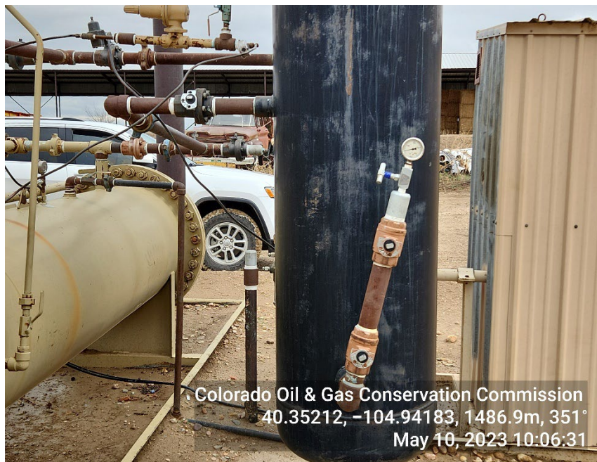
Photo 7: Valve appears to be open, pressure present on gauge
