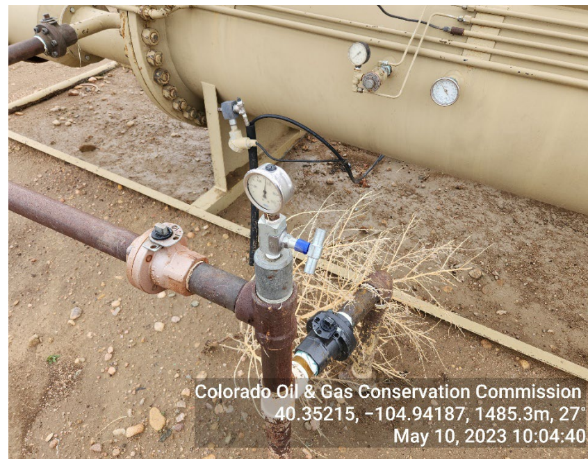
Photo 4: Valves appear to be open
