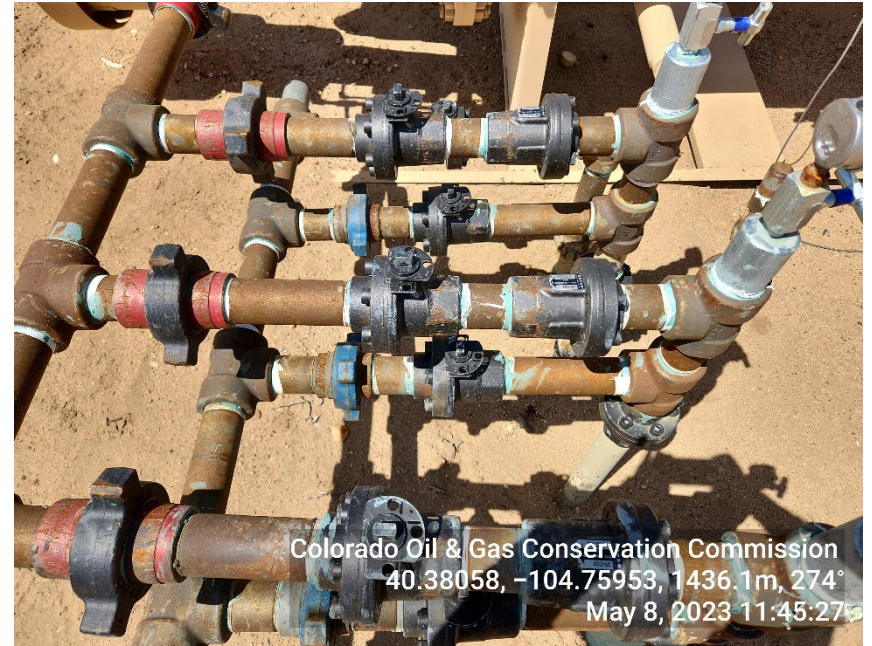
Photo 8: Valve appears to be open
