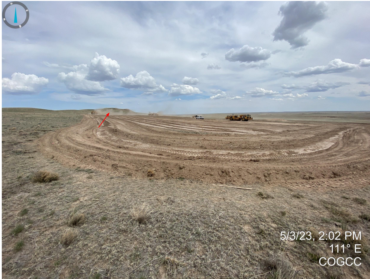
Photo 5. Facing east from the northwest corner of the pad construction. Photo illustrates topsoil salvage operations and fugitive dust (red arrow) that was observed at the time of this inspection. Also pictured, a temporary stormwater BMP (ditch and berm) appears to have been installed during the construction phase of the location.
