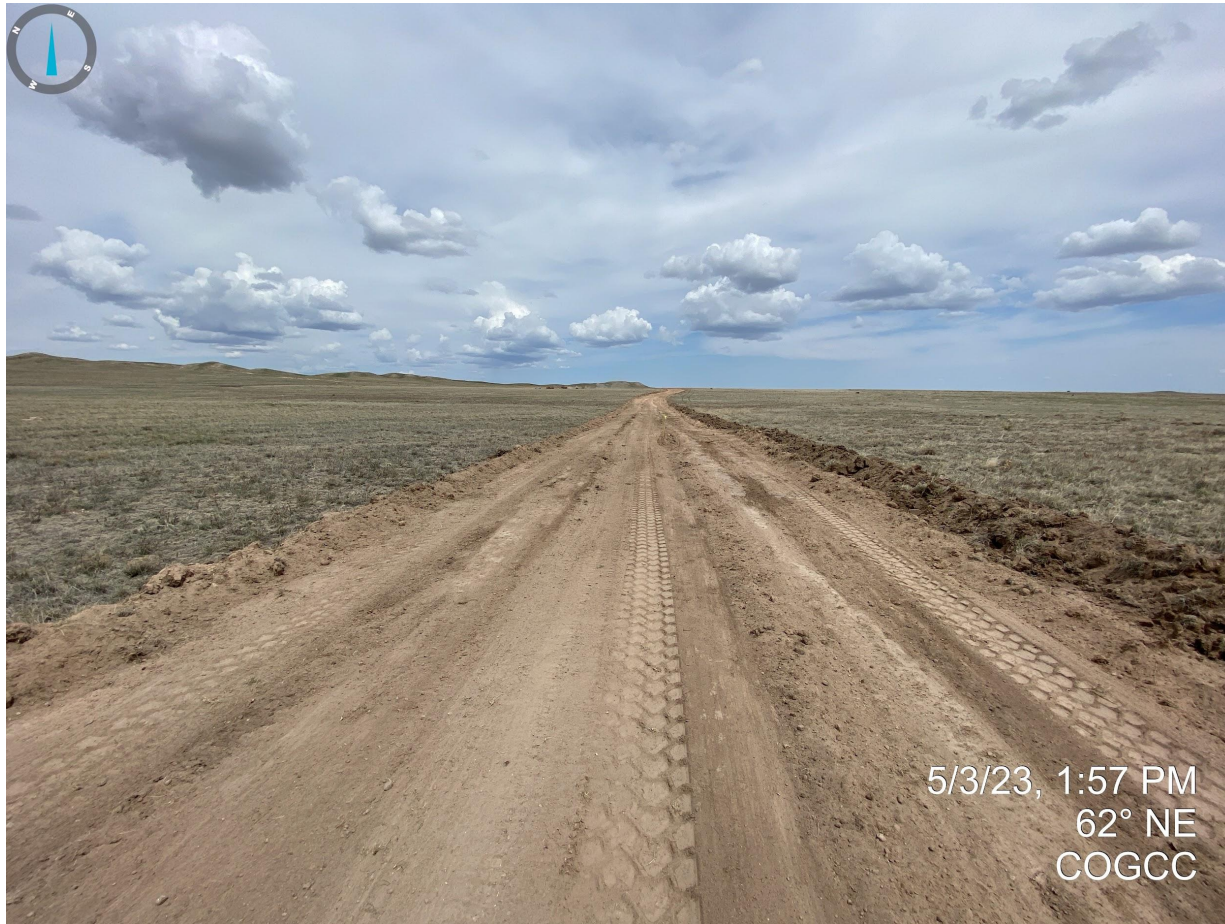
Photo 4. Facing northeast from an existing access road. The access road appears to have been grubbed and widened during the construction process.
