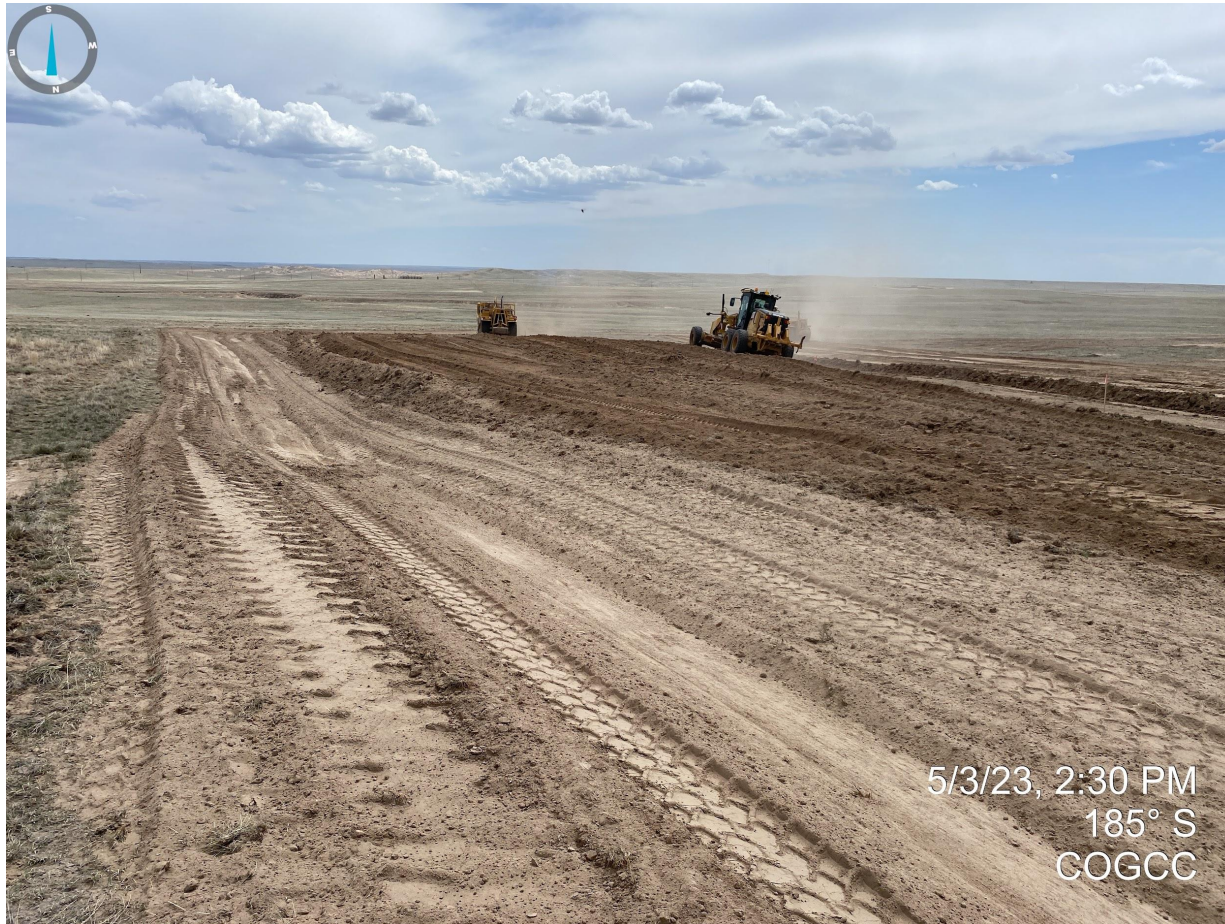
Photo 8. Facing south towards the topsoil stockpile. A future inspection will be conducted to ensure all topsoil has been salvaged from the location and that stockpiles are stabilized against wind and water erosion.
