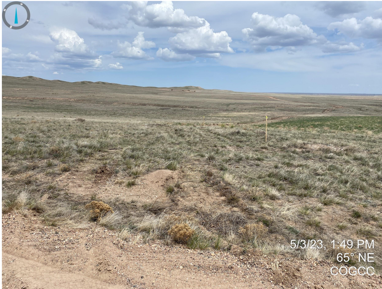
Photo 1. Facing northeast from the new access road entrance. At the time of this inspection, it did not appear topsoil had been salvaged from the access road with evidence of some grubbing having occurred. An approved copy of the From 2A was also not posted on location at the time of this inspection.
