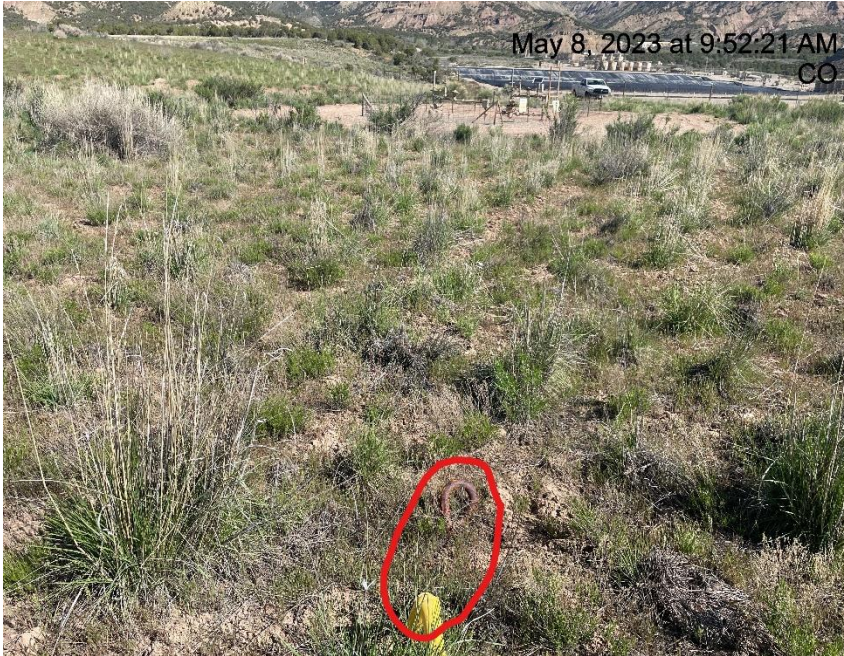
Photo # 7207 Improperly marked deadman
